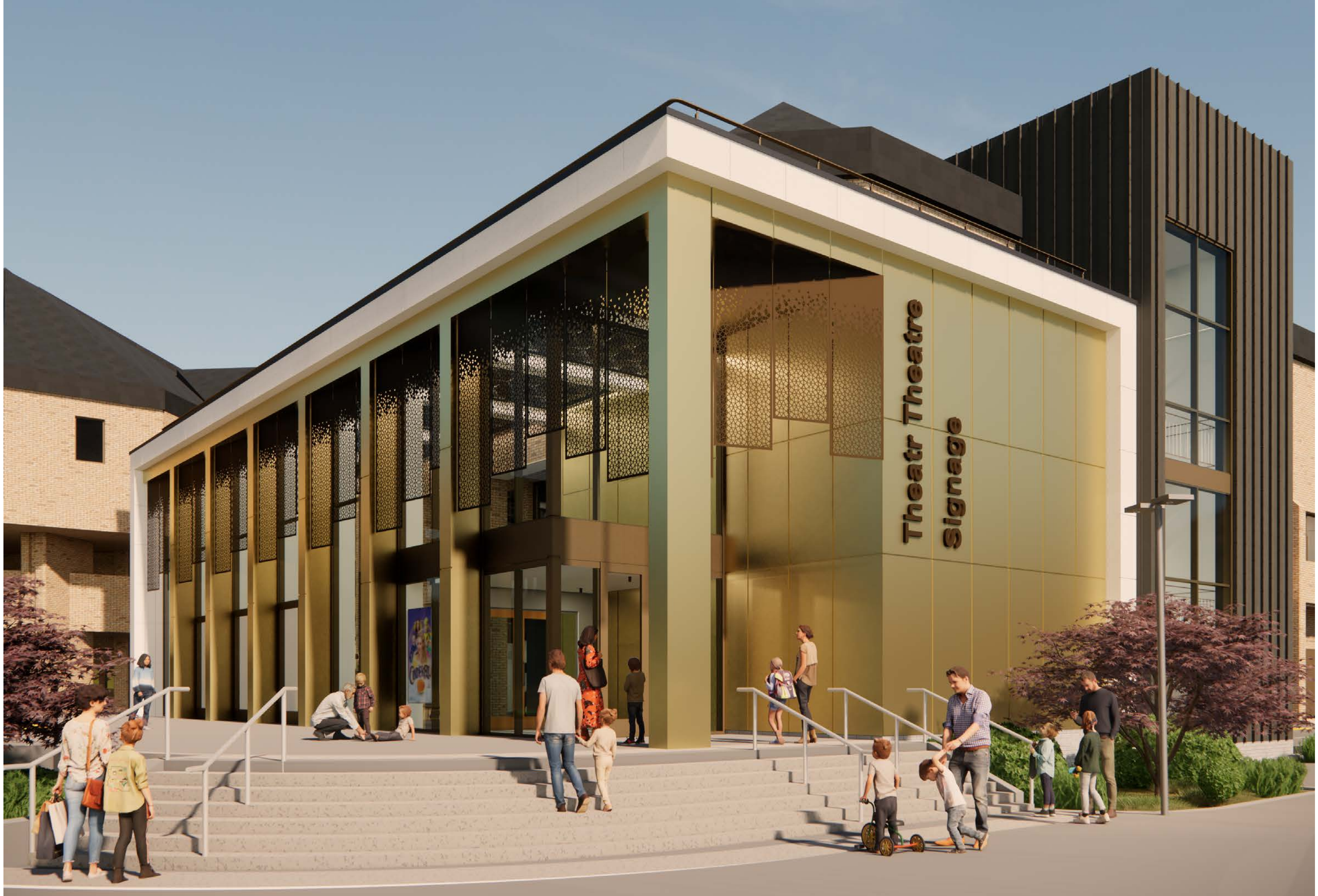
View of the main entrance with the civic centre in the background
