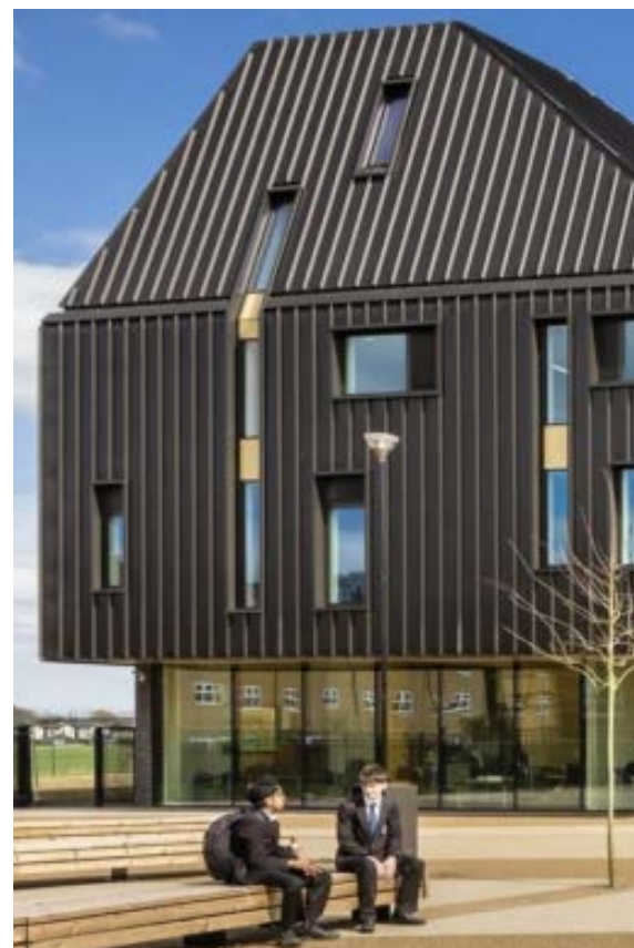
04 Standing Seam Cladding PPC aluminium (colour: anthracite)
