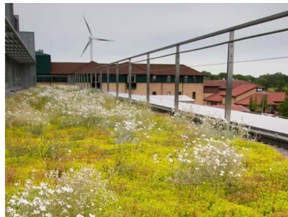
11 Extensive Green Roof and PPC Roof Guarding
