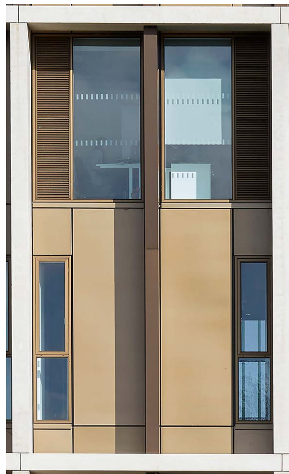
02 Aluminium Cladding Anodised Aluminium (colour: Regency Gold)
