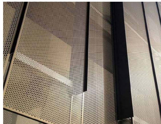
03 Perforated Brise Soleil Screens Anodised Aluminium (colour: Dark Umber, Anolok 545)
