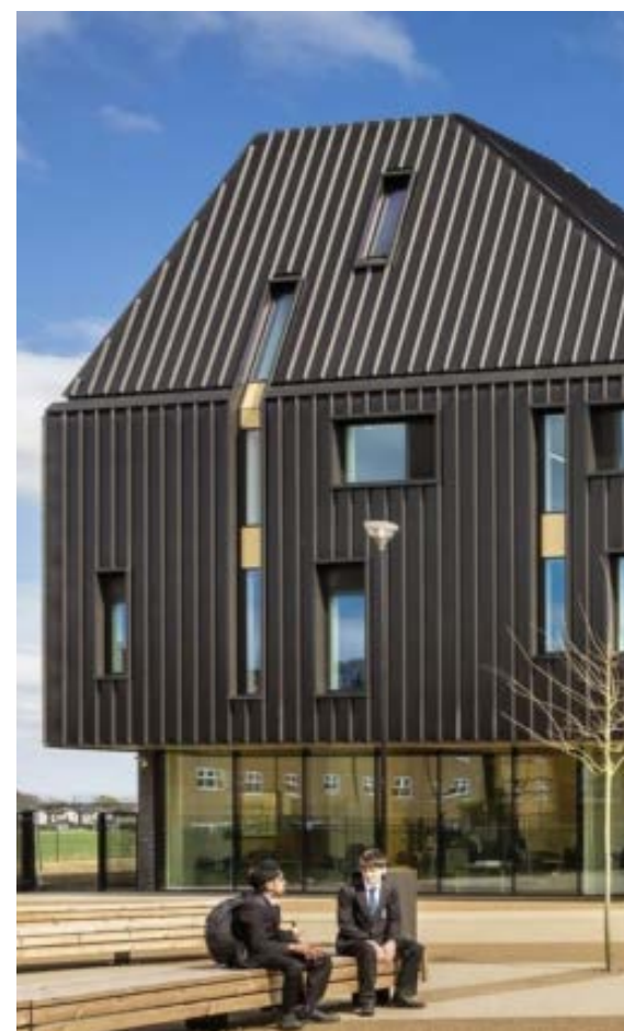
04 Standing Seam Cladding PPC aluminium (colour: anthracite)
