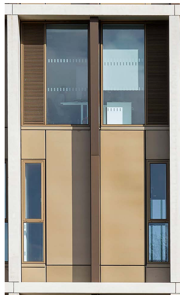
02 Aluminium Cladding Anodised Aluminium (colour: Regency Gold)
