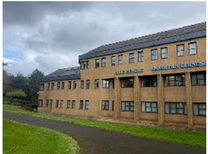
North west view of building
