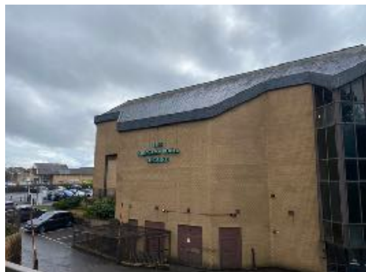
North east view of building
