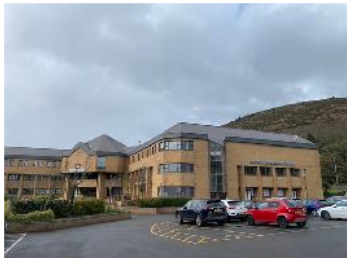
South east view of building
