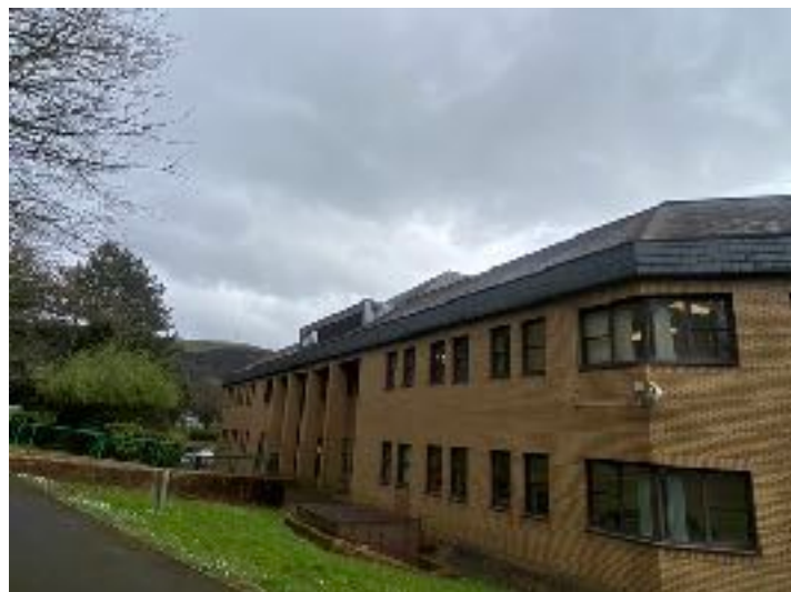
North view of building
