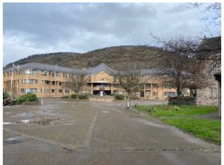
Paved area to south of building
