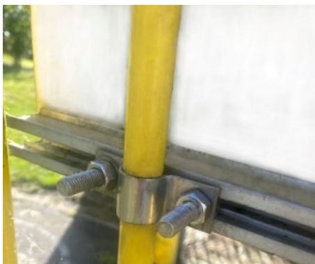
Photograph 4 – Back view of proposed fixing method
