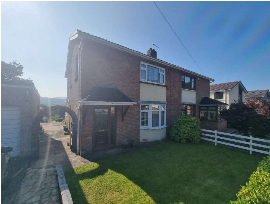
Front elevation view including front lawn area and concrete driveway
