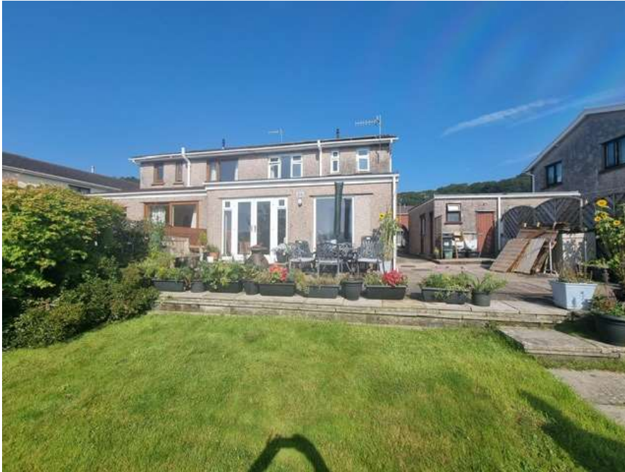
View of rear elevation including lawn and outbuilding/garage to be demolished
