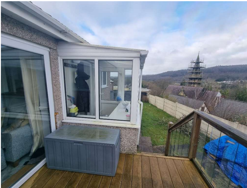
Existing raised decking area
