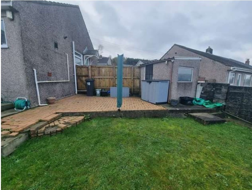
Rear lawn area, blockwork wall to neighbours side and some outbuildings
