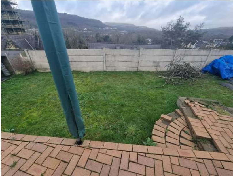
View of rear boundary concrete panel wall and lawned area
