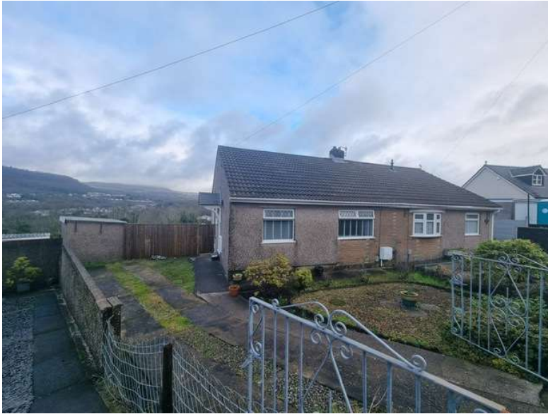
Front elevation view including front yard area and driveway
