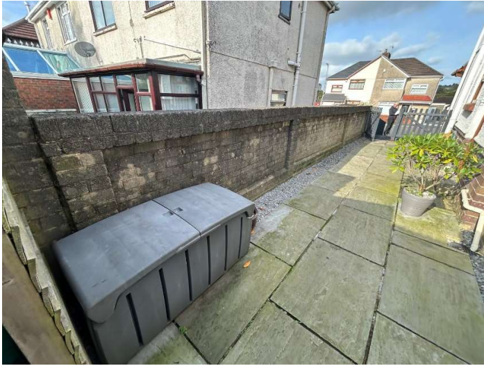
Side boundary view of brickwork boundary wall
