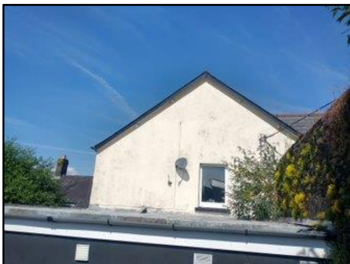
Photograph 4. Main building North elevation.
