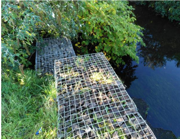
Figure 15 - View of the feeder from the road bridge showing Japanese knotweed.
