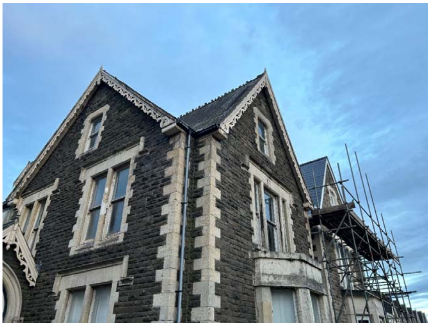
Plate 2 Surveyor view to north western corner.
