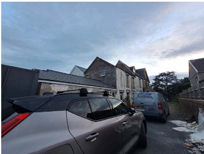
Plate 1 Surveyor view to northern elevation.
