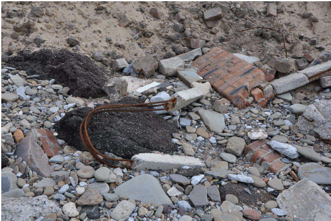
Plate 6 (4396) – Tarmac, Concrete, Steel and Masonry from Eroding Cliff.
