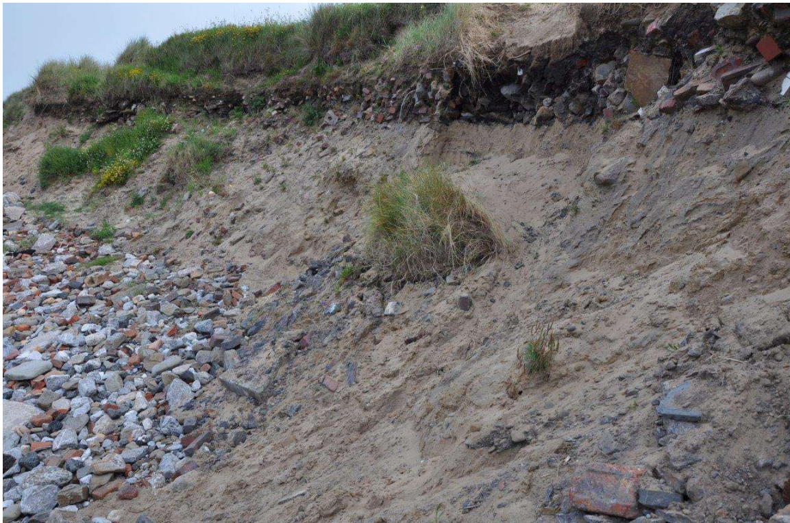
Plate 17 (4426) – Eroding Cliff / Recession Pocket and Band of Demolition Material.
