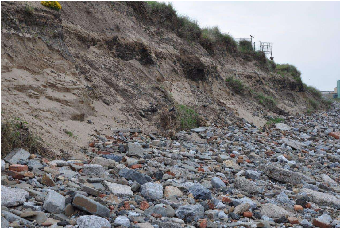
Plate 12 - (4402) – Eroding Cliff – Note the band of debris part way up face and composition of storm beach.
