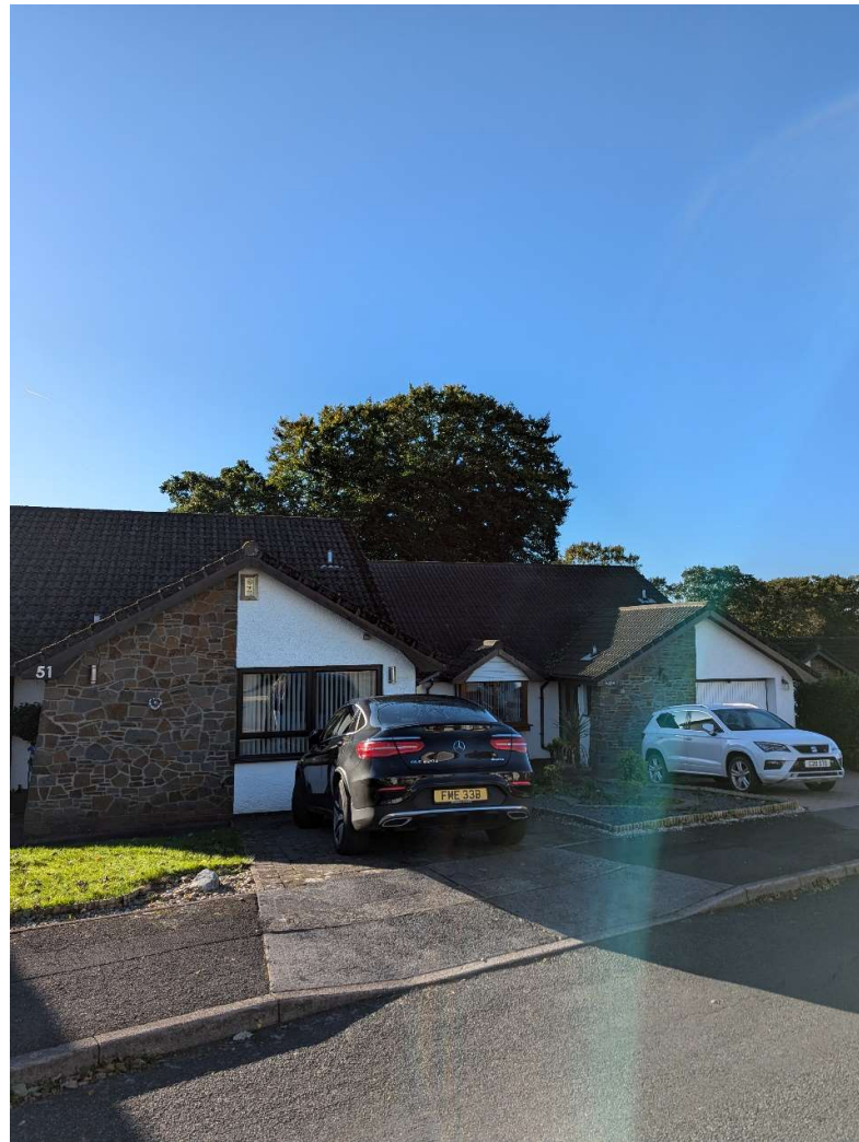
Figure 6 View from Daphane Road over 51 & 49
