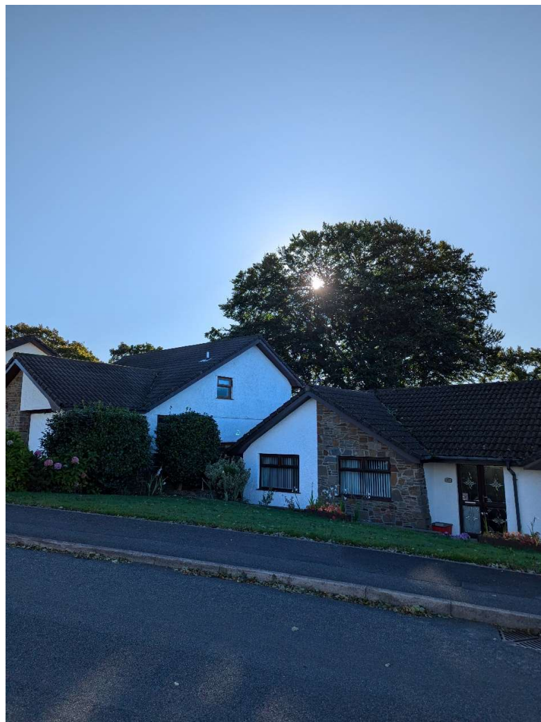
Figure 4 View from Daphne Road over 47 & 49
