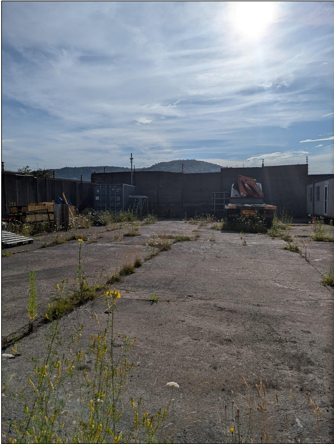
Plate 7: The enclosed yard near the middle of site.
