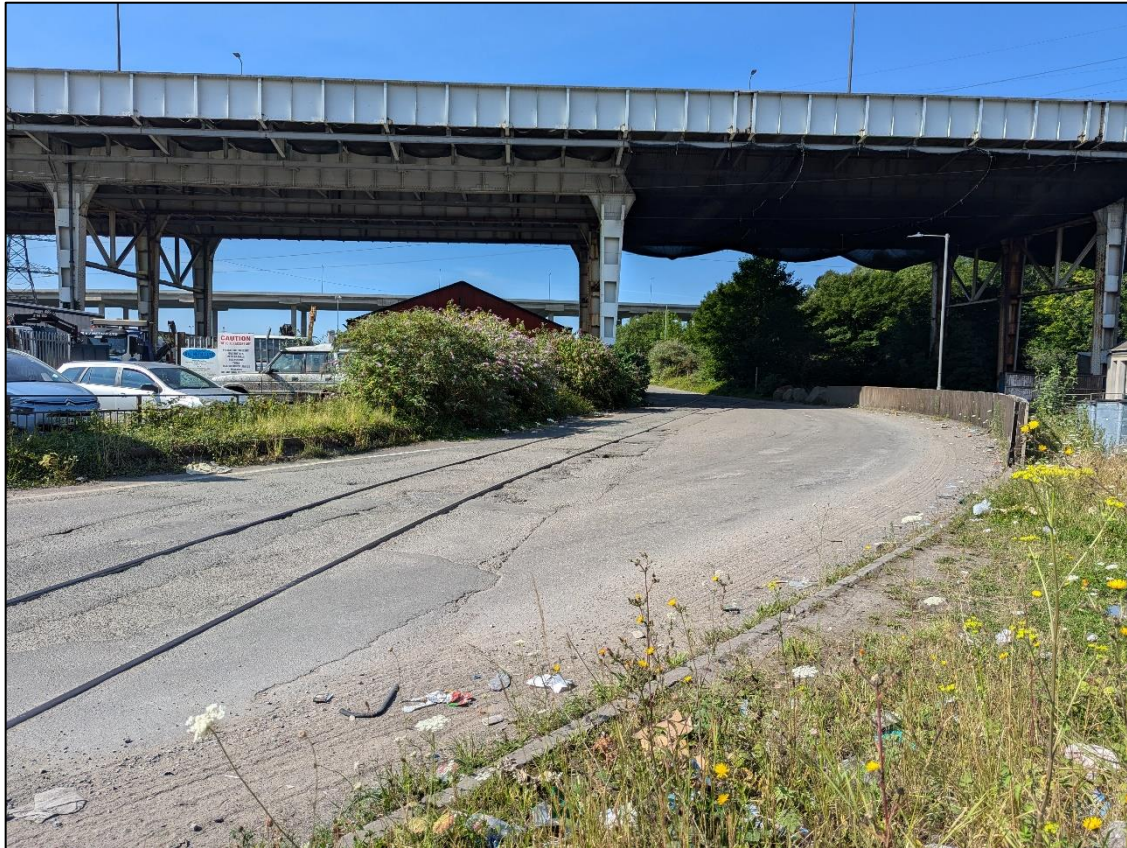
Plate 1: Railway lines on approach to site.
