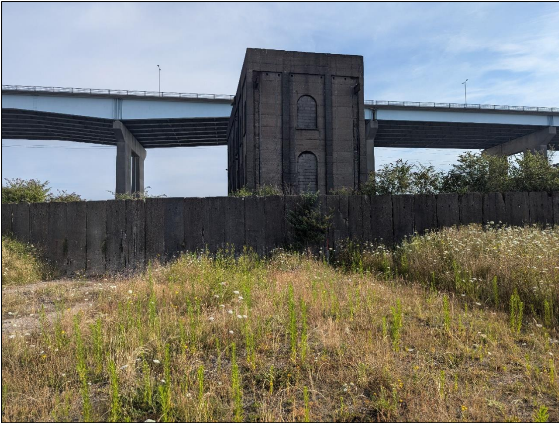
Plate 3. View north of the Briton Ferry Ironworks Engine House and M4 viaduct.
