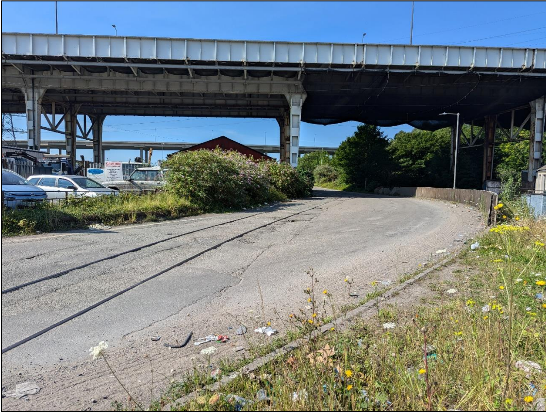
Plate 1: Railway lines on approach to site.
