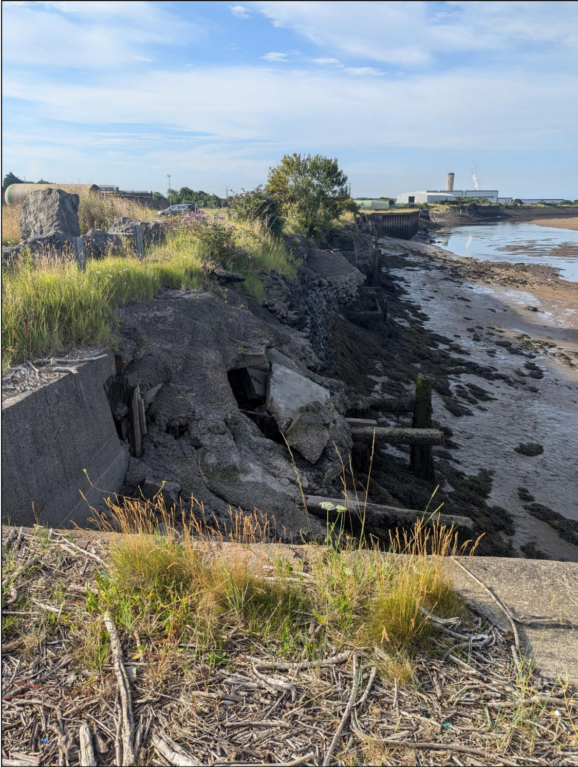
Plate 4. View south along wharf.
