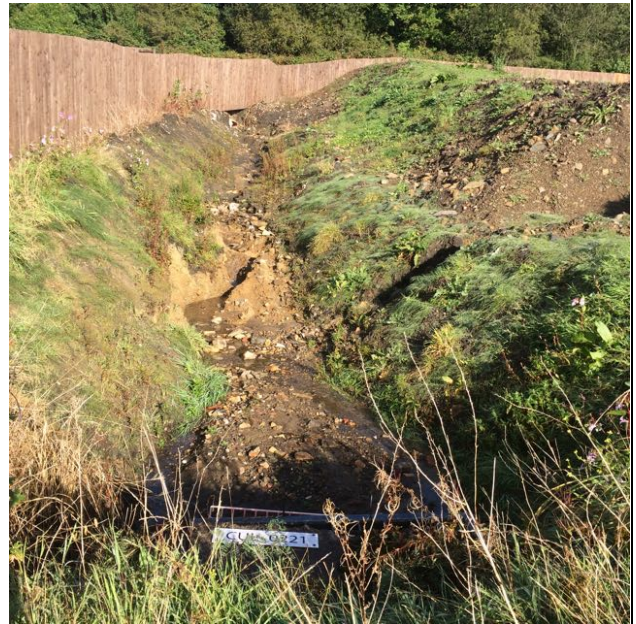
Figure 4. Drainage ditch along western boundary.
