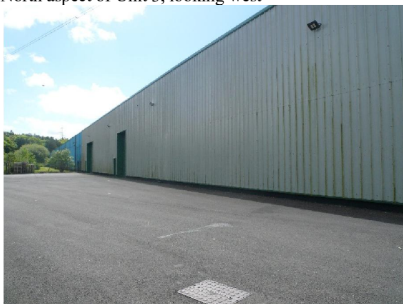
North-east aspect of Unit 3, looking south-east
