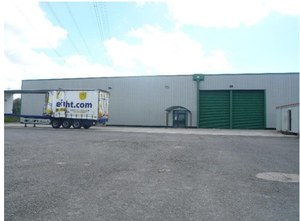
North-west aspect of Unit 3, looking south-east
