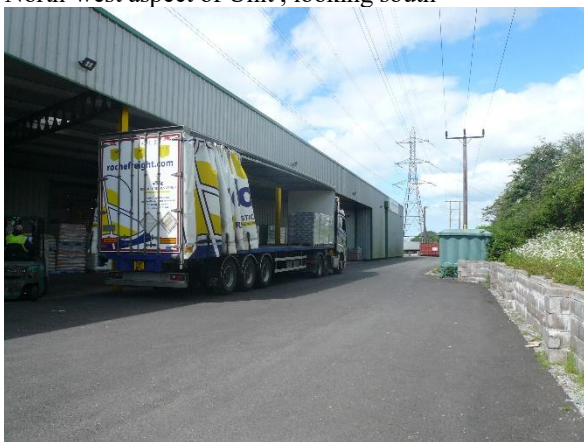
North aspect of Unit 3, looking west
