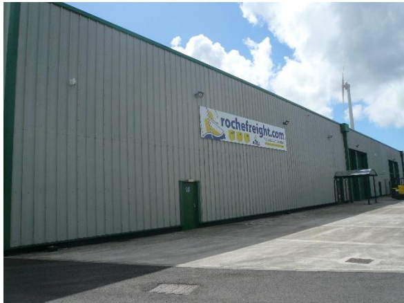
North-west aspect of Unit 3, looking south
