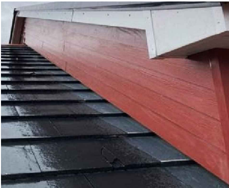
Hardie Plank Cedral cladding to stepped gable - on-site image
