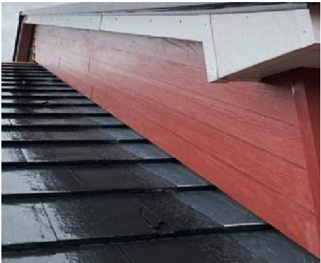
Hardie Plank Cedar cladding to stepped gable - on-site image
