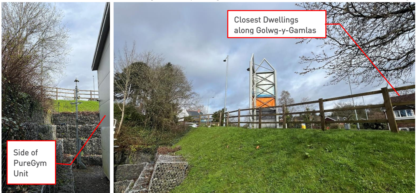
Figure 4 – Separating Embankment between Pure Gym demise & Dwellings
