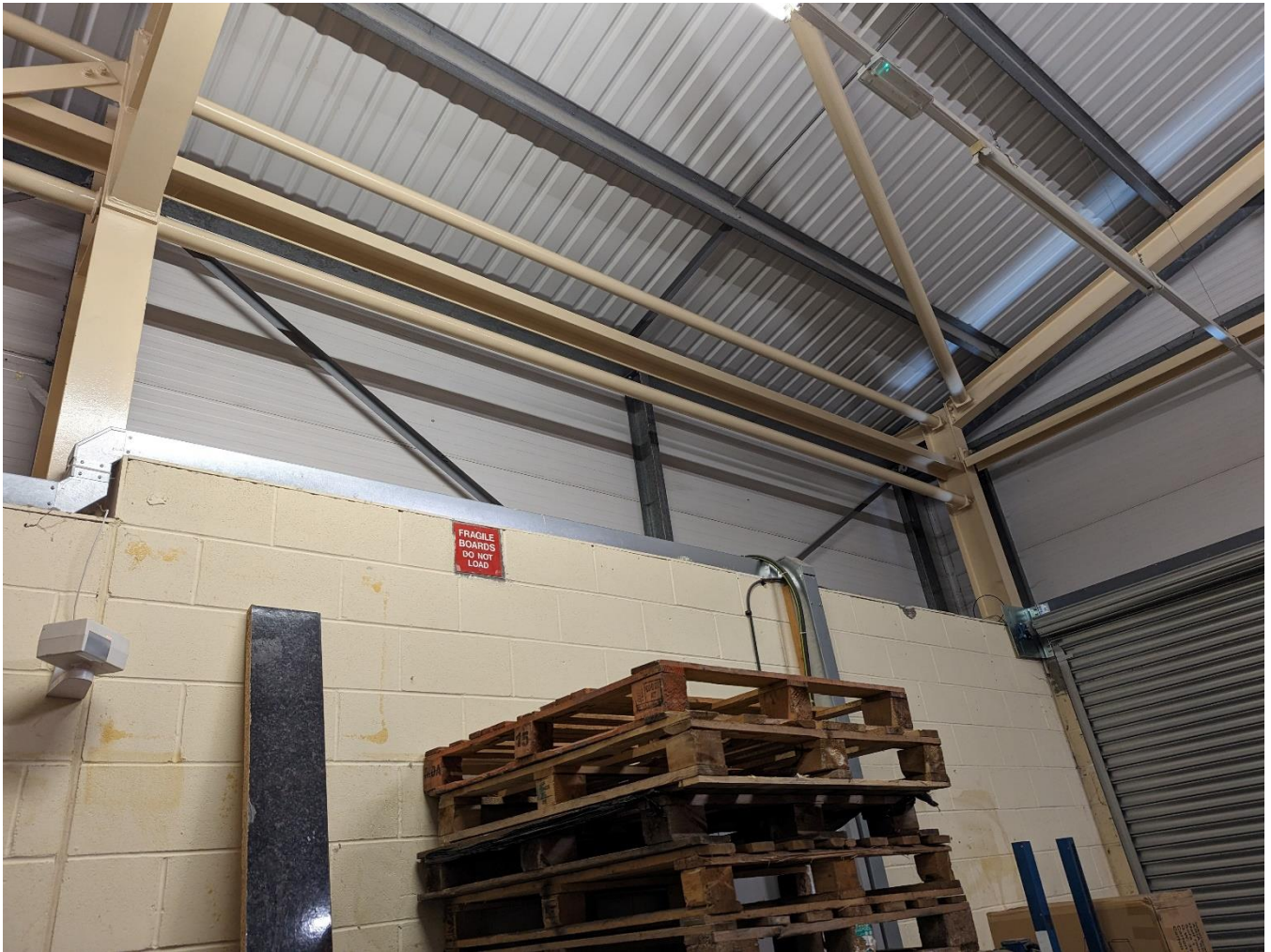
Figure 2 – External Façade Constructions II
