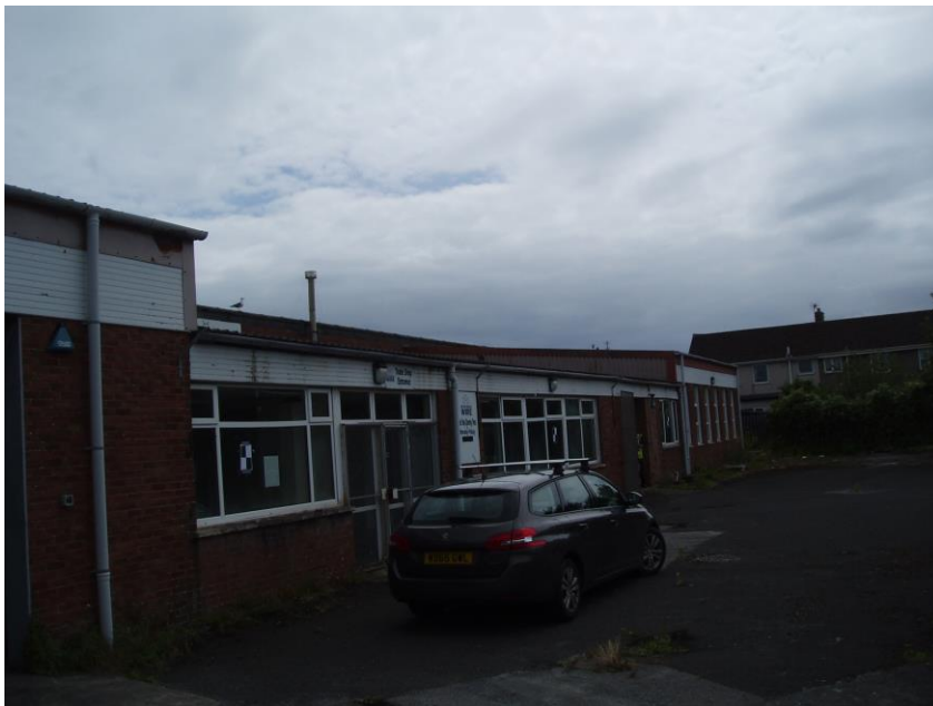
The front extension looking east.
