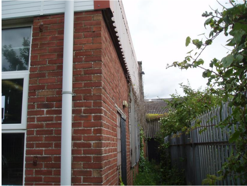
The eastern end of the office block with the main unit to the rear
