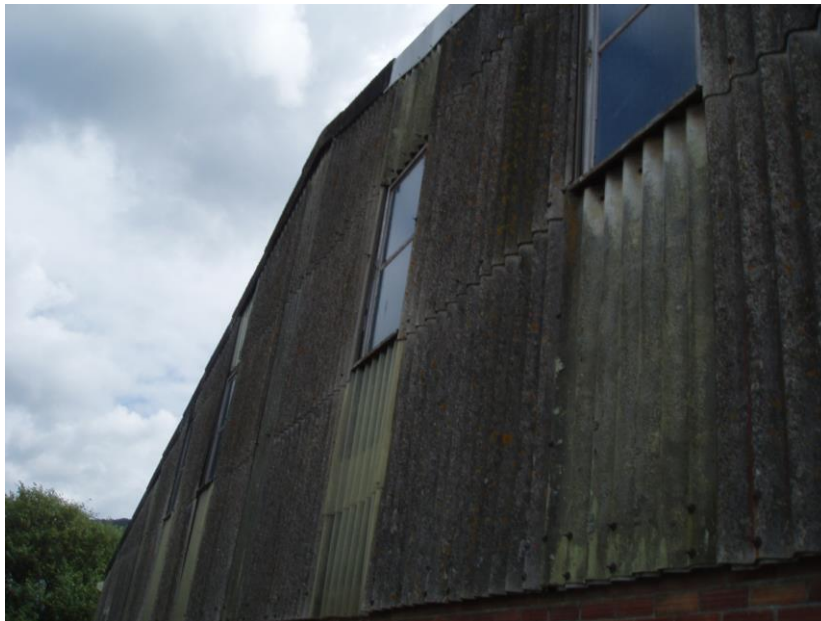
Views of the eastern elevation showing single storey brick wall (top) with cladding above (lower)
