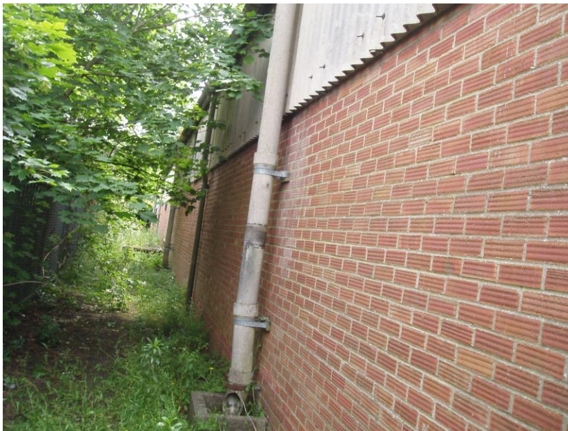
The rear of the property (adjacent to Afan Way)
