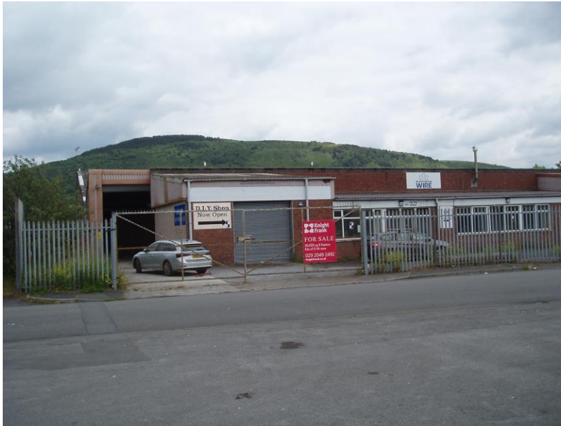
The front elevation on Acacia Avenue
