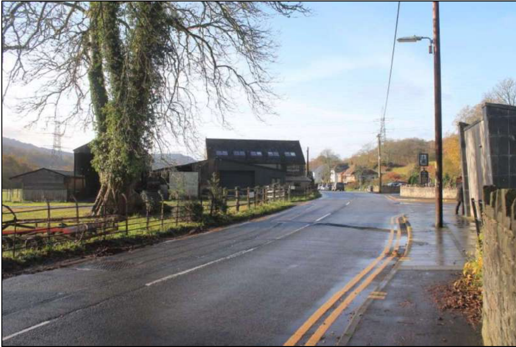
Photo 4: View southwest towards the proposed development area from the main road as it crosses the adjacent bridge. The agricultural buildings and roof of Sgwyd Gwladys is visible on the left.
