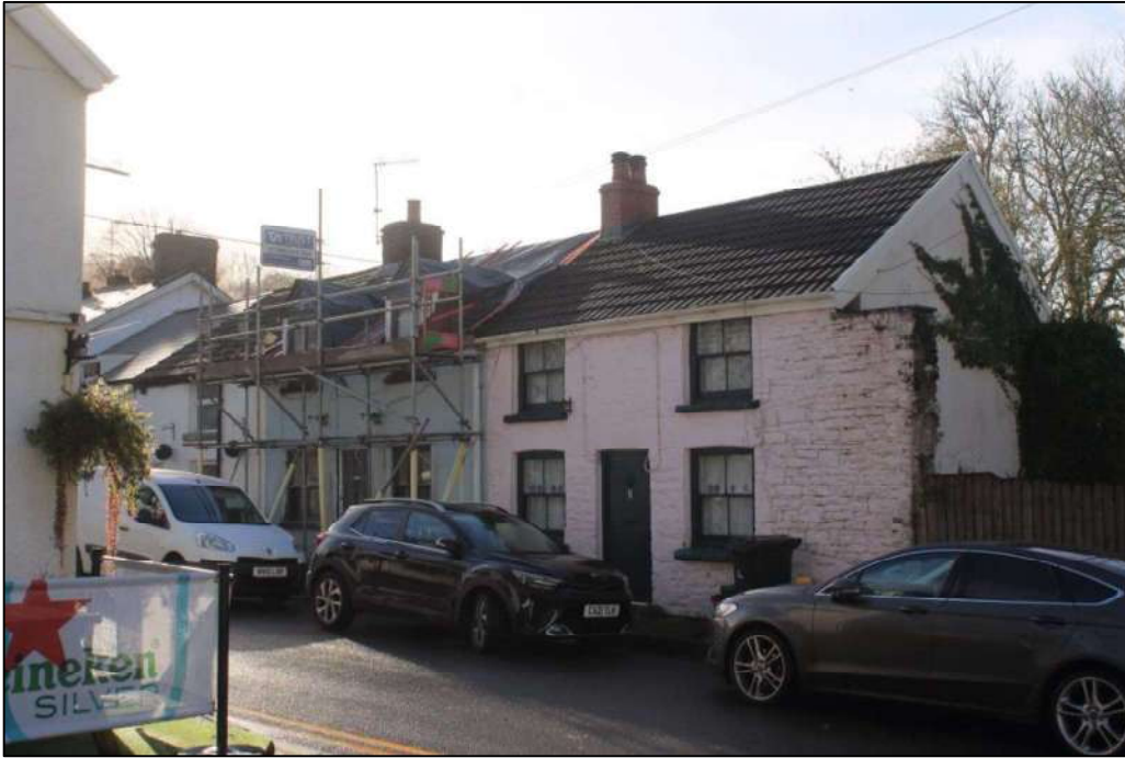
Photo 20: View north showing the traditional buildings fronting High Street on the east side of the river.
