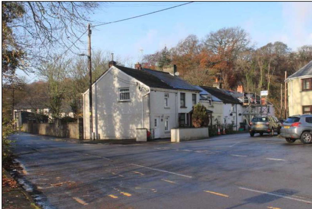
Photo 19: View northwest showing the traditional buildings fronting High Street on the east side of the river.
