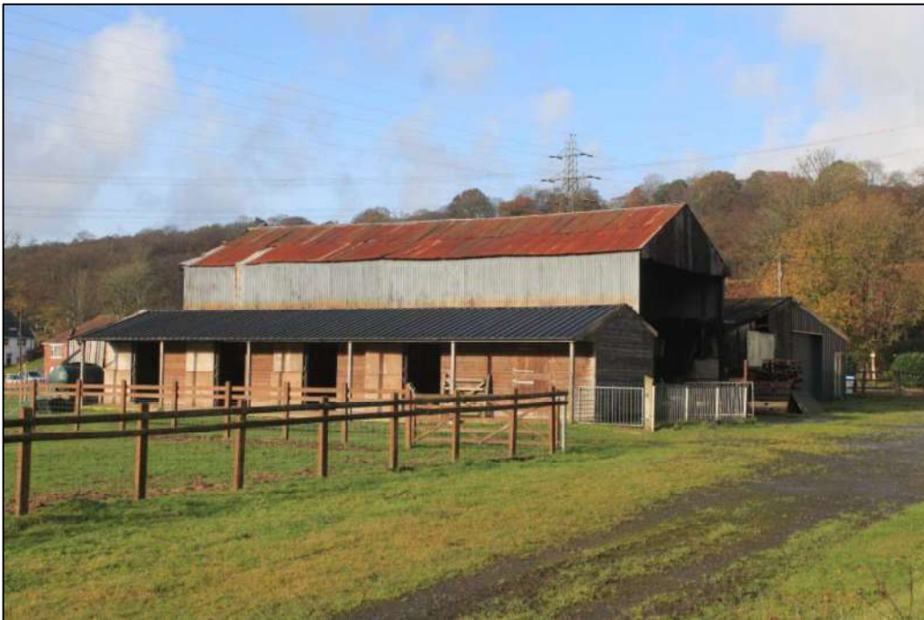
Photo 9: View northwest showing the agricultural buildings within the proposed development area.
