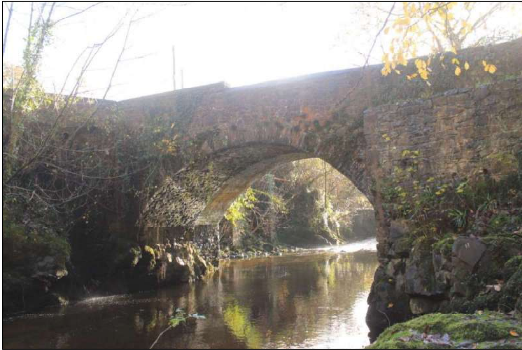
Photo 16: View southeast showing the old bridge (NPRN 24139) in Pontneddfechan.
