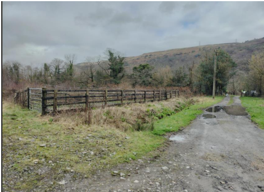
Figure 5, Photo of existing menage, looking east towards the access
