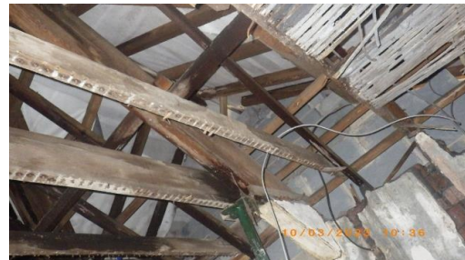
Roof timbers and tarpaulin over section A
