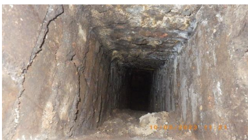
Remains of chimney stack in section B
