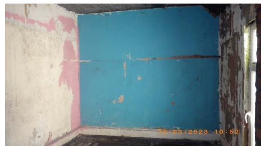
Section A to the rear side of the property
