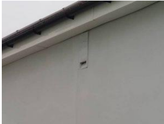
Bat Tube integrated into design of house
