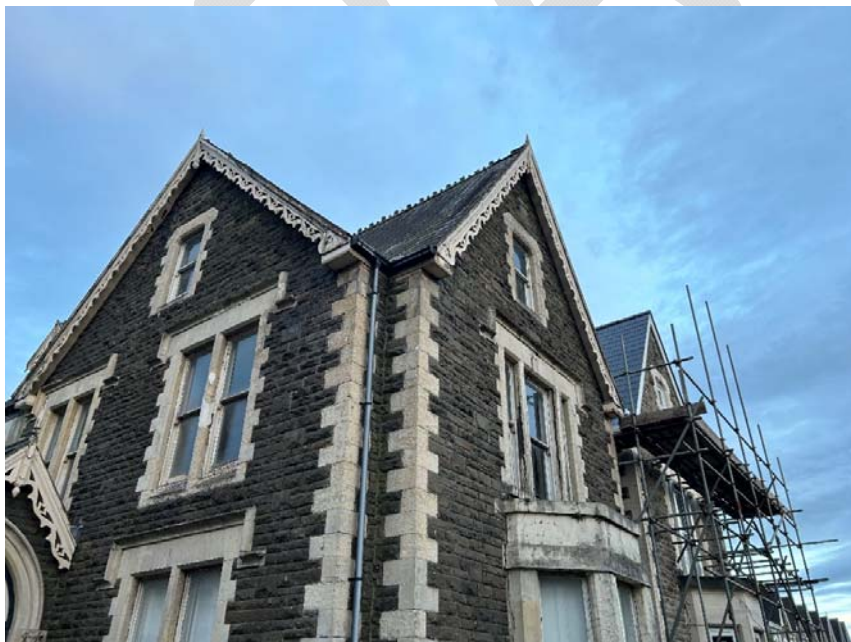
Plate 2 Surveyor view to north western corner.
