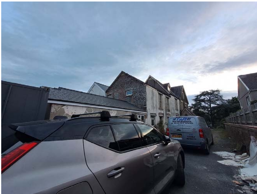
Plate 1 Surveyor view to northern elevation.
