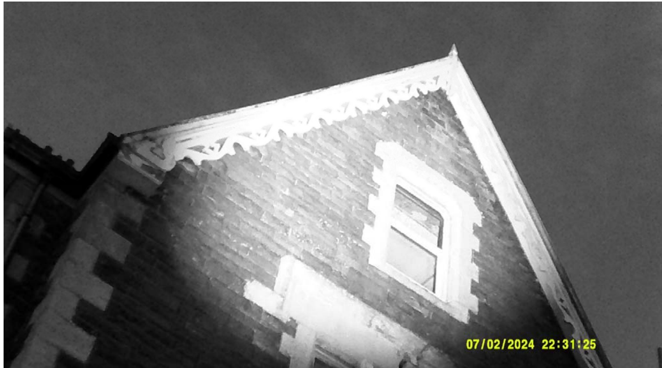
Plate 3 Night Fox Image of western gable, 22.30h
