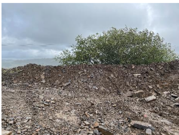
View of location of end of exposed pipe which has been removed and no visible flow of water.
