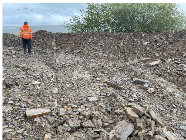
View of former path of exposed pipe that has been removed and no visible water, looking towards W21 which is located beyond the bund.
