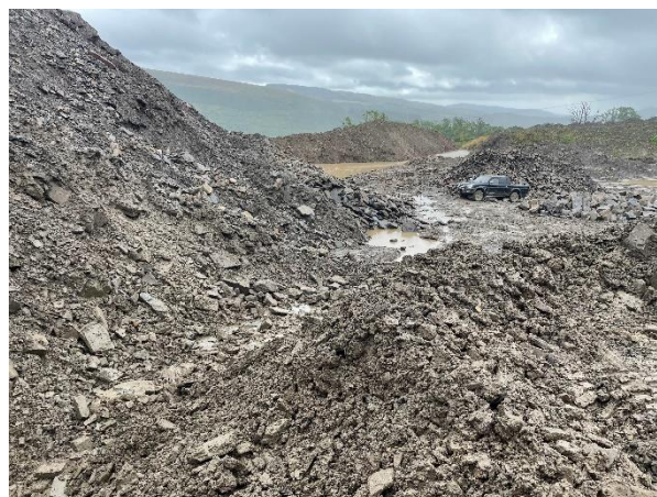
Looking SE at water flow of quarry surface water along western side of tip down gradient into quarry sump.
