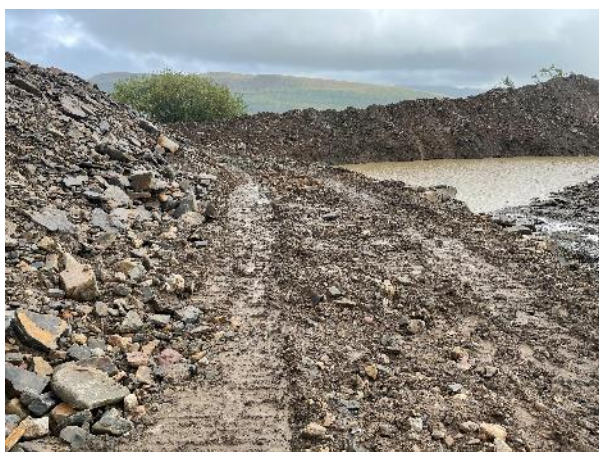
View of former path of exposed pipe that has been removed and no visible flow of water.
