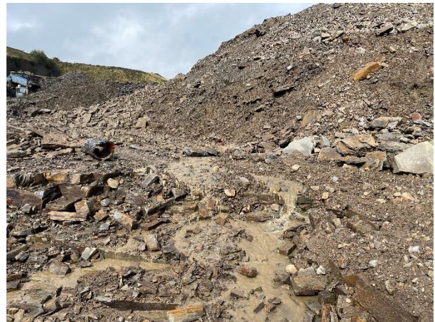
Looking towards end of pipe beneath tip with water flowing down gradient over bedrock towards the SE into the quarry sump.
