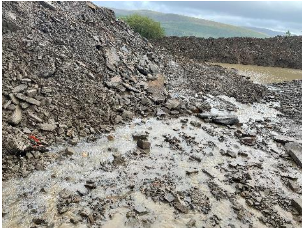
View of point where quarry surface water from west of tip meets water from pipe and flows into quarry sump.
