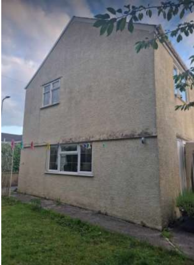
Plate 1- Photograph of gable that extension is to be attached
