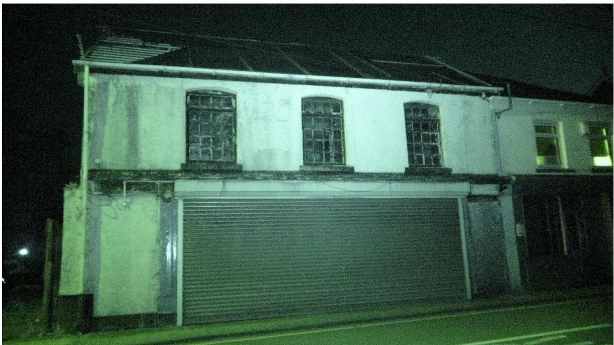
Photograph of the north east elevation of the property at the darkest point of the survey
