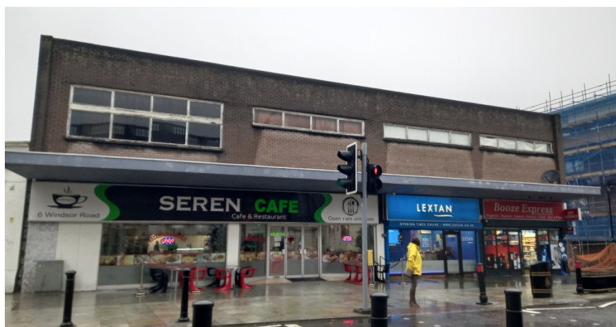
Front of the site
