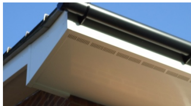
White soffit boards to roof overhangs
