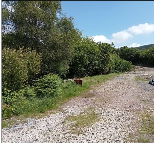
Site from entrance North Boundary
