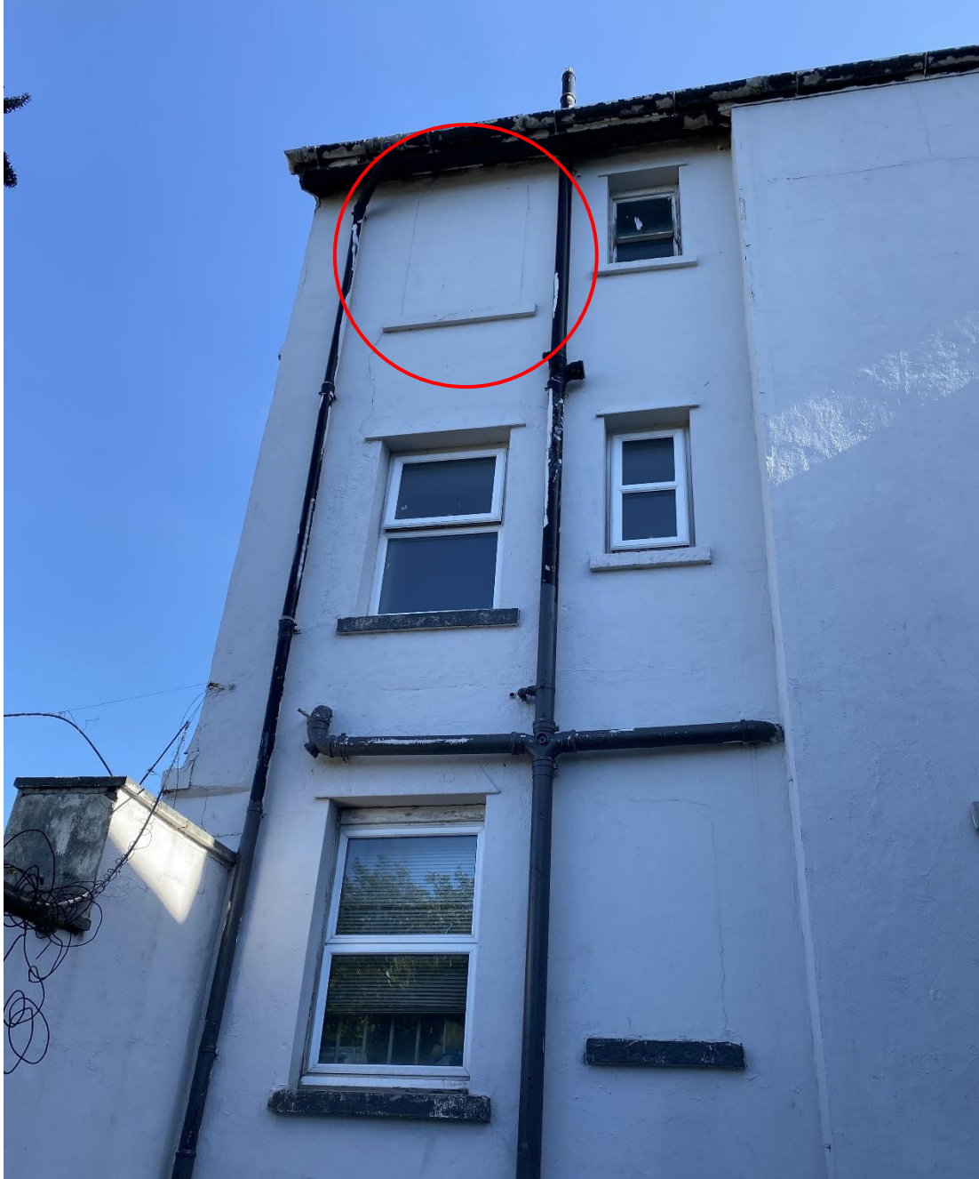
Figure 23: Photograph showing the existing blocked up second-floor window (highlighted by the red circle) which is proposed to be reinstated as part of the proposed works – refer to LBA drawing 0526_P04.
