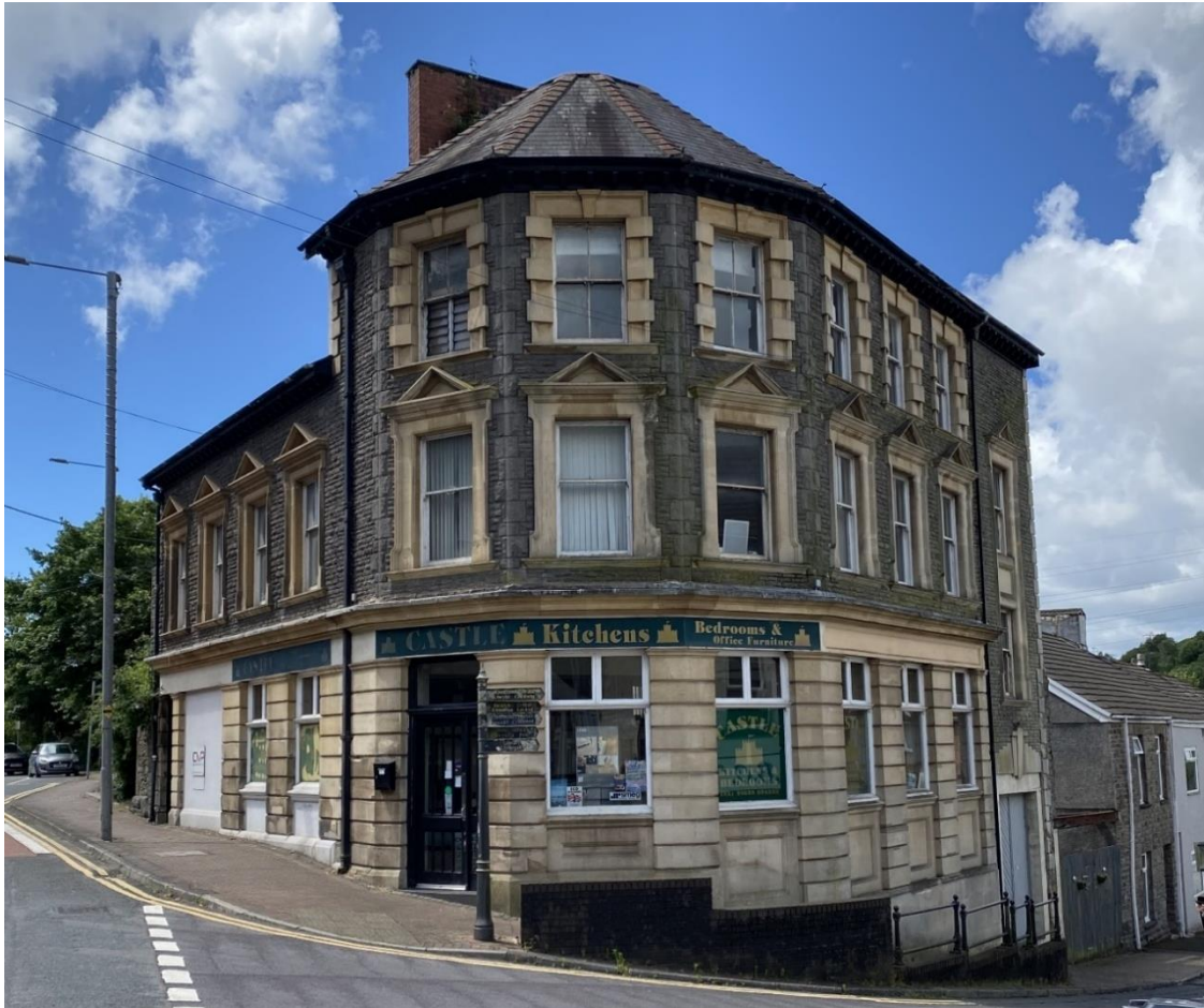
Figure 09: Photograph showing the prominent corner elevation of 43, Neath Road – with Neath Road to the left and Villiers Street falling away to the right. The property is designated as a Building of Local Importance (Ref. BFE001) as a “ Well preserved building of character that forms a noticeable feature in the streetscape and provides evidence of Briton Ferry’s past commercial importance. Group value with former bank (Listed Building) and Post Office (BFE018) on opposite side of Neath Road ”.
