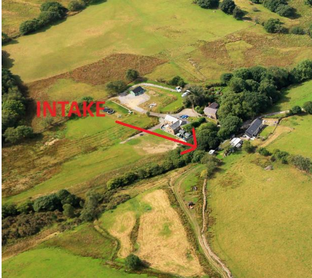
Intake Location Photo
