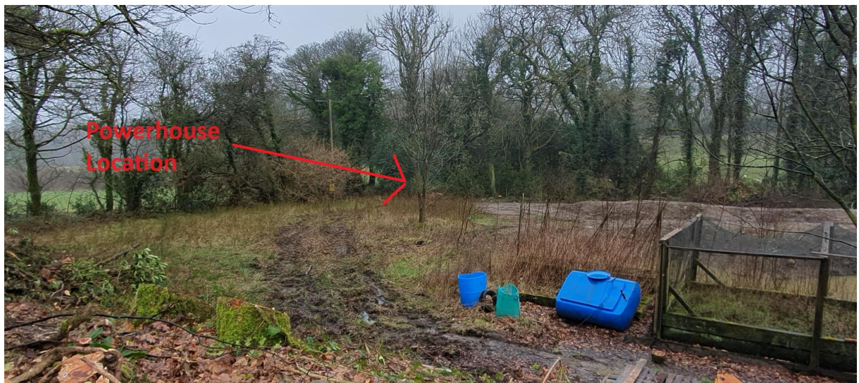
Powerhouse Location (photo taken looking West)
