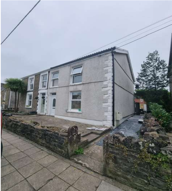
Front elevation view showing small yard area
