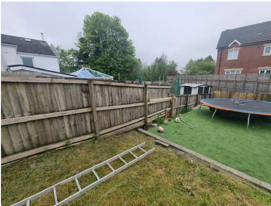
View of adjoining neighbours boundary
