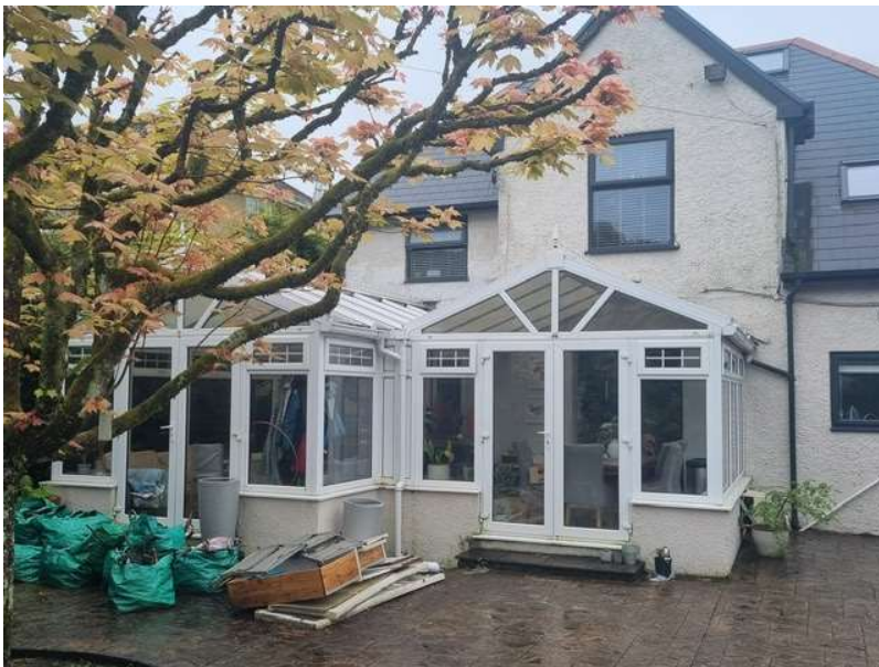
Photo of existing rear extension where the replacement extension will be sited and the enlarged infill area will be erected on the existing patio area
