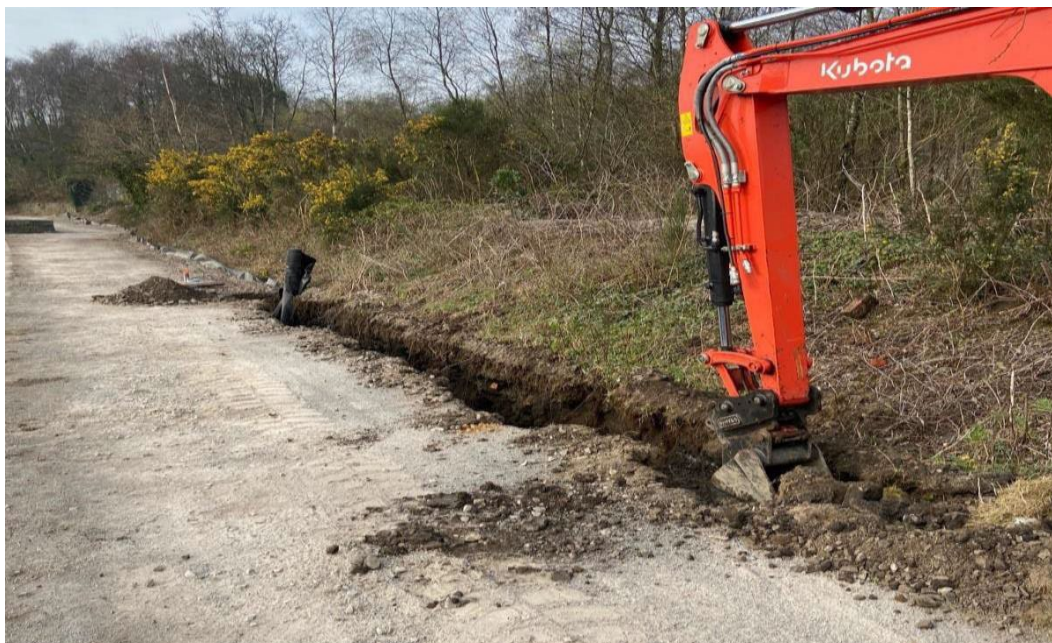
CSK installing 2.5m deep JK barrier membrane in Swansea to protect a new footpath
