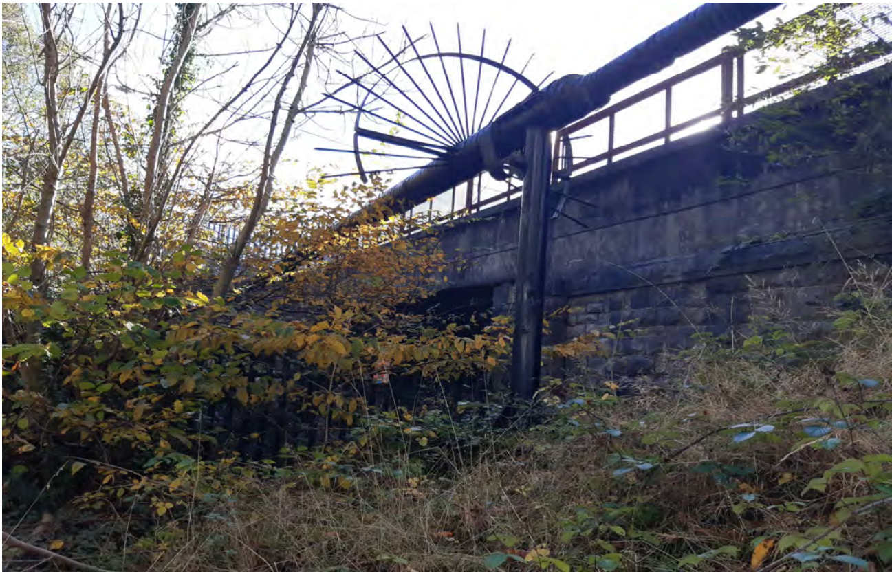
9 - Above ground gas pipe to south of site (looking southeast)
