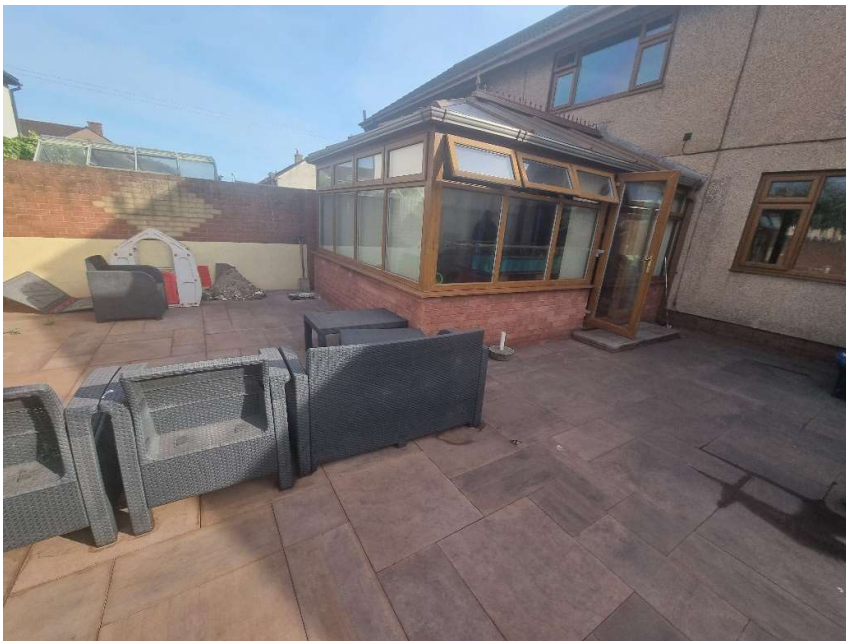
Existing extension which is to be replaced and brickwork wall to neighbours boundary
