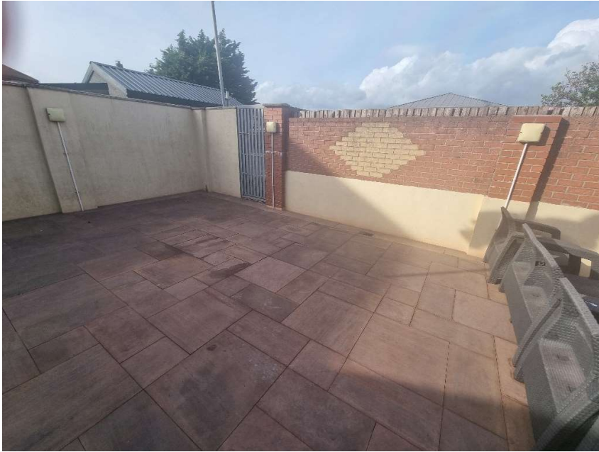
Rear brickwork/blockwork wall and paved patio area
