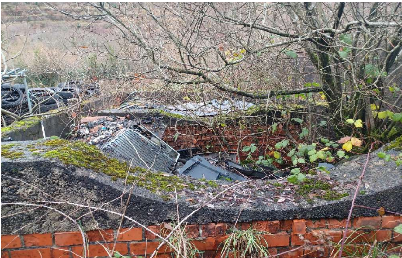
39 Water tank housing (no tank remains)
