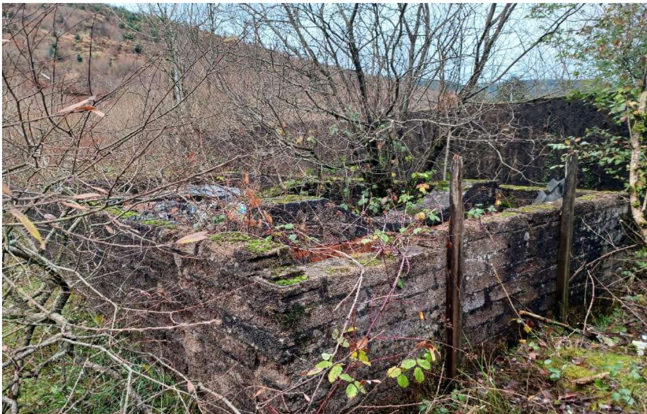
38 Water tank housing (no tank remains)
