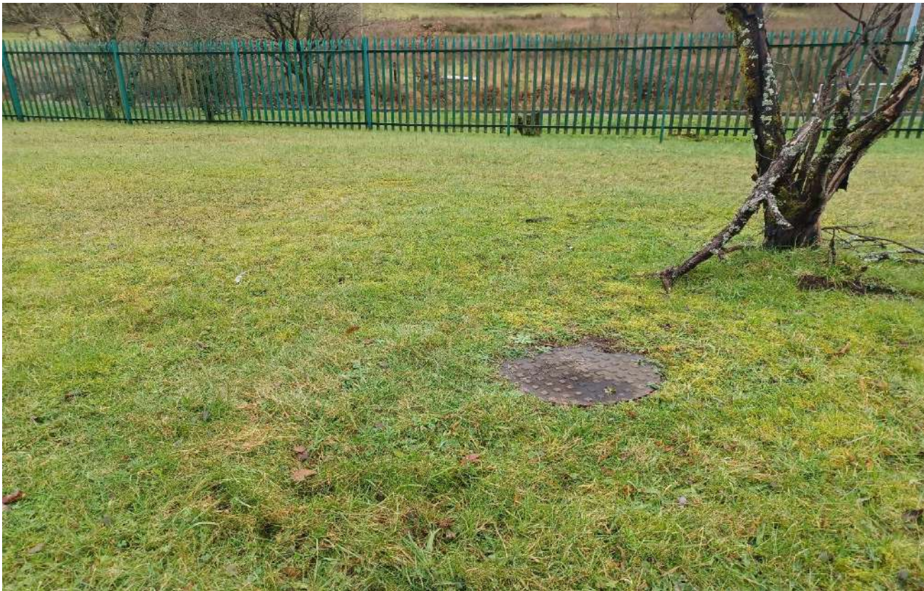
35 Manhole in grass towards S corner
