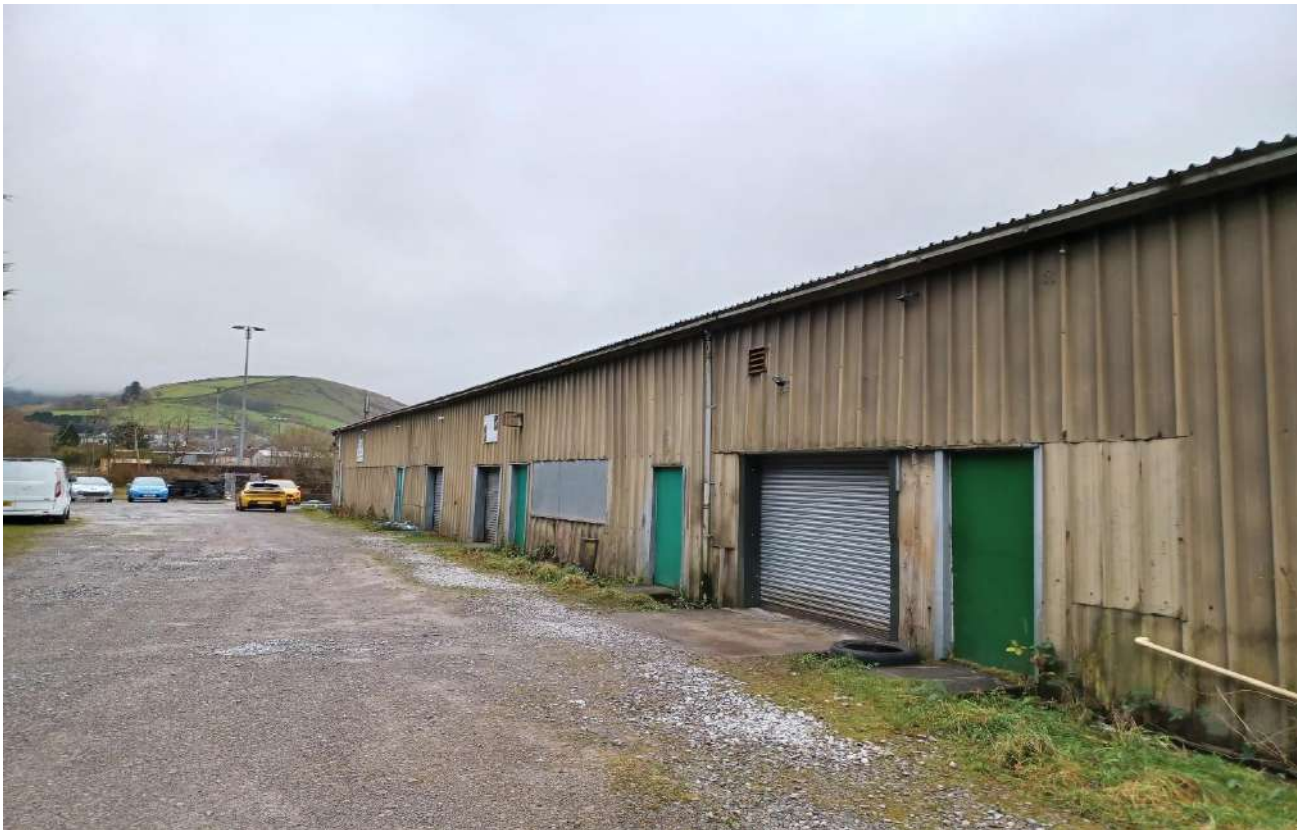
9 Behind existing workshops (facing E)
