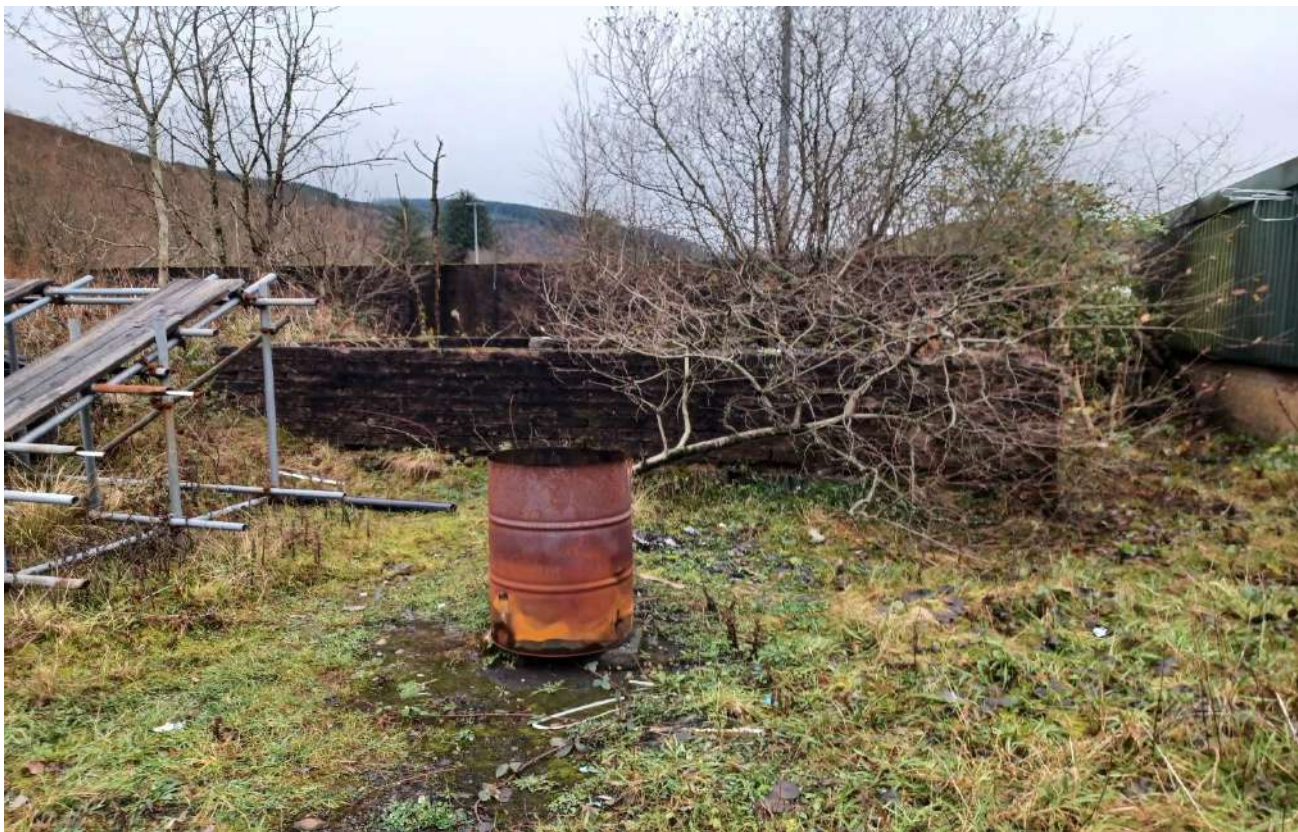
37 Water tank housing (no tank remains)
