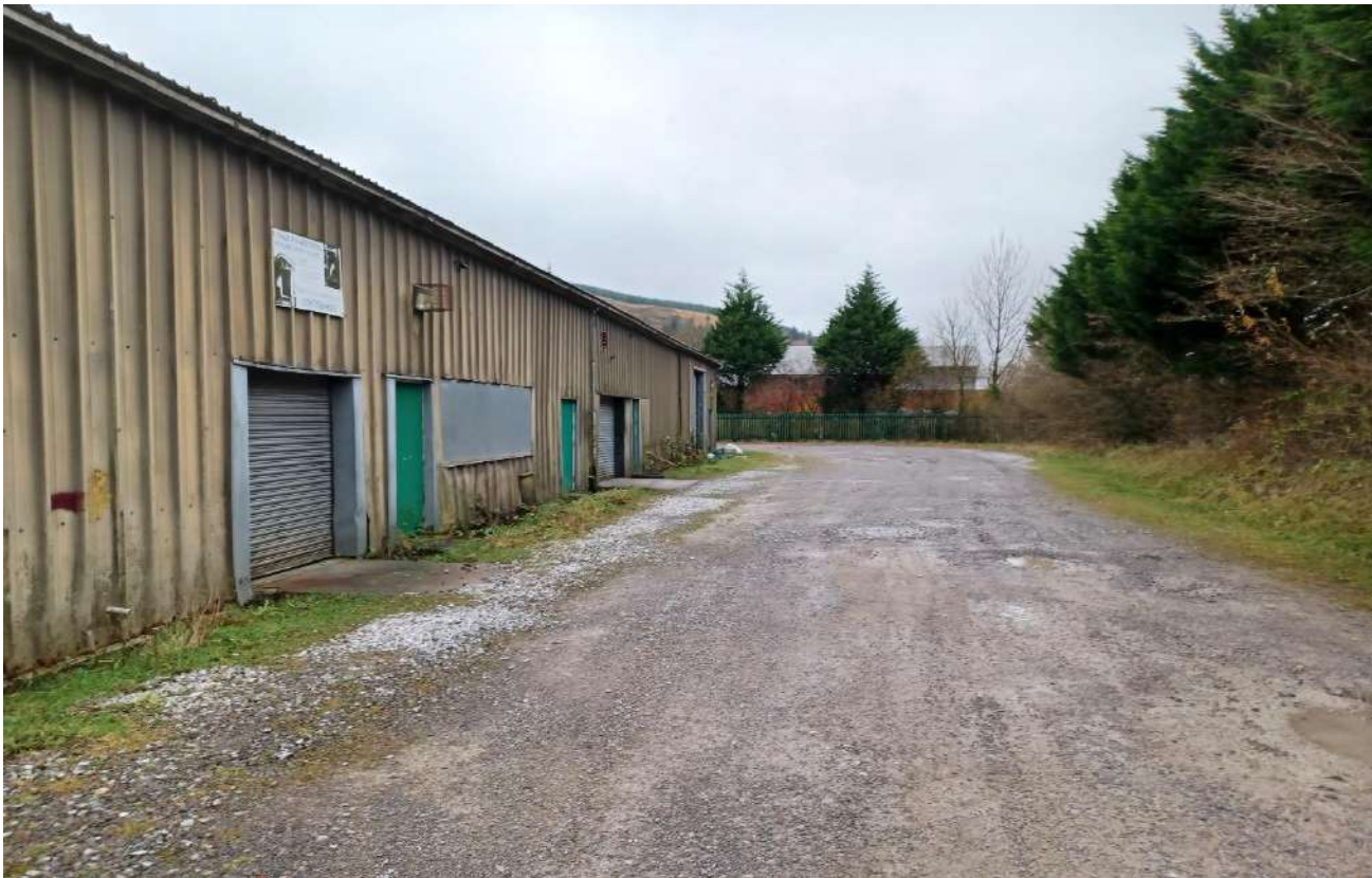
10 Behind existing workshops (facing SW)
