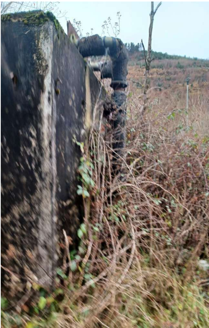
15 Pipeline to dismantled building (view from behind small workshop)
