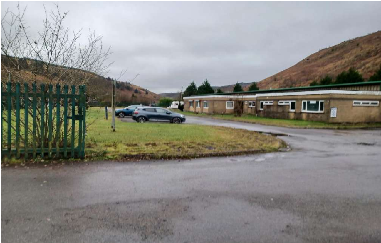
22 Glyncorrwg workshops (view from entrance facing SW)
