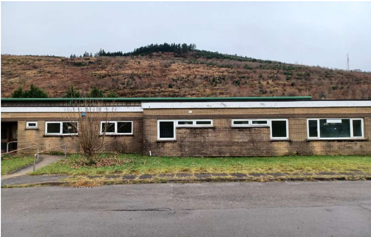
25 Existing workshops (facing NW)
