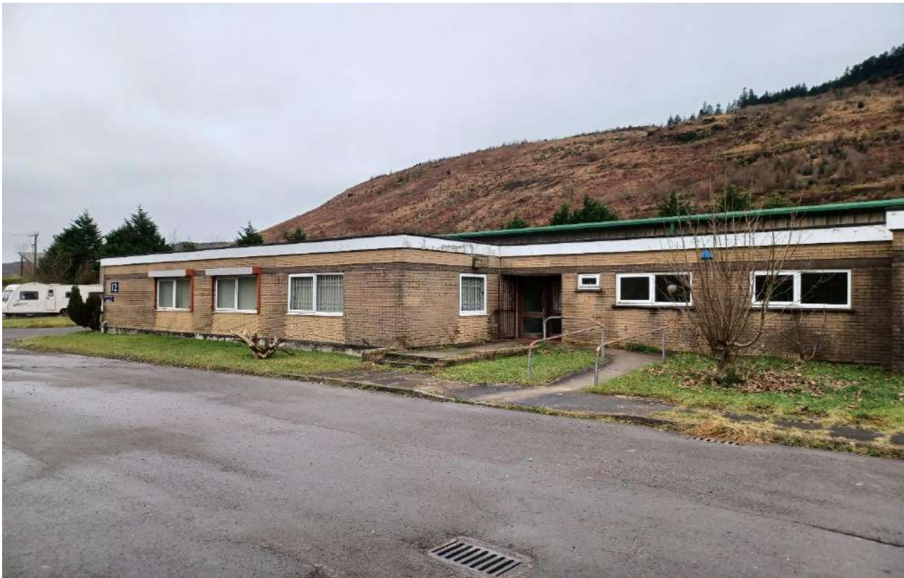
26 Existing workshop building (facing W)
