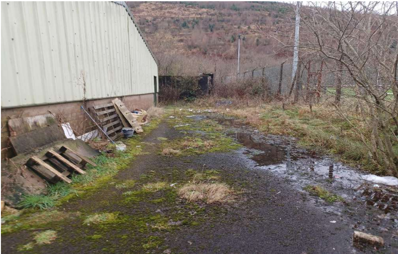
13 Behind smaller workshop (facing NW)
