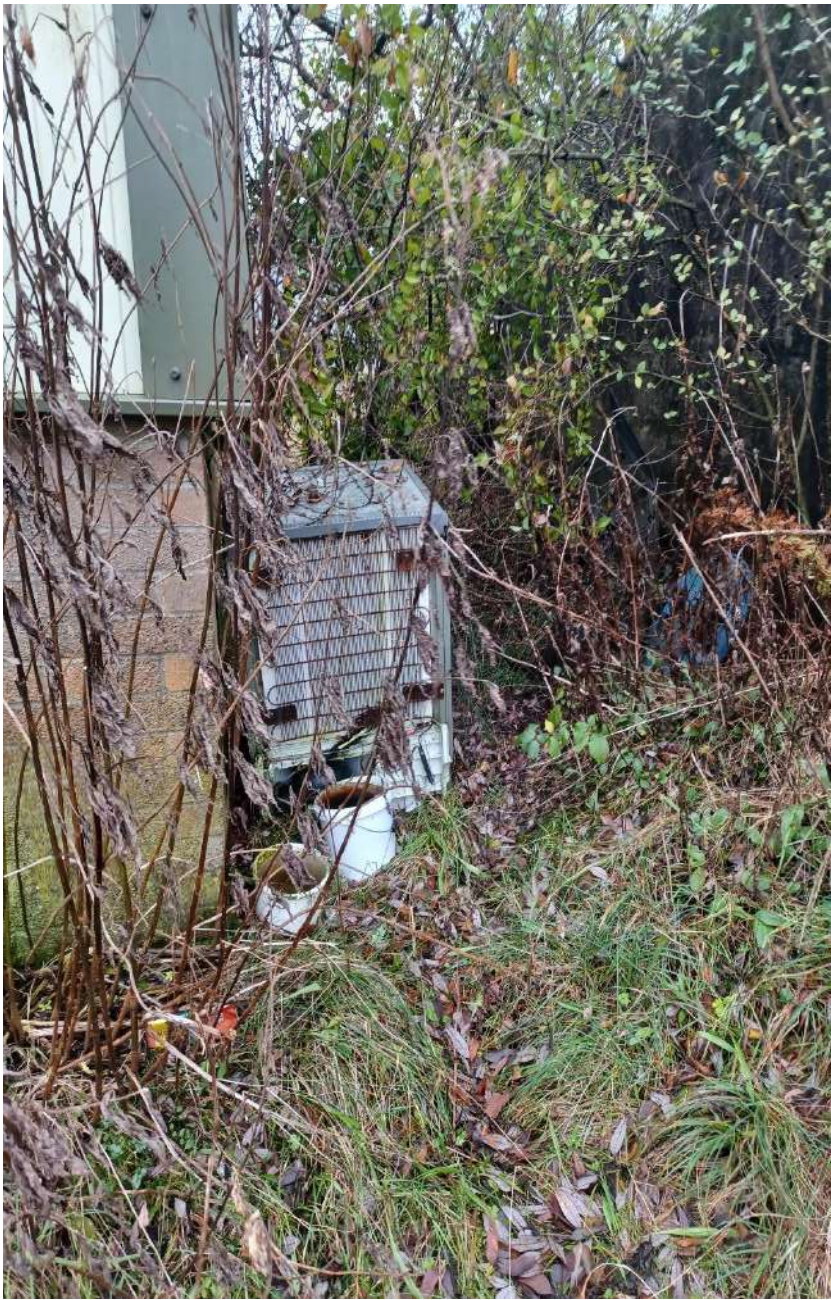
16 Flytipping behind small workshop (facing SW)
