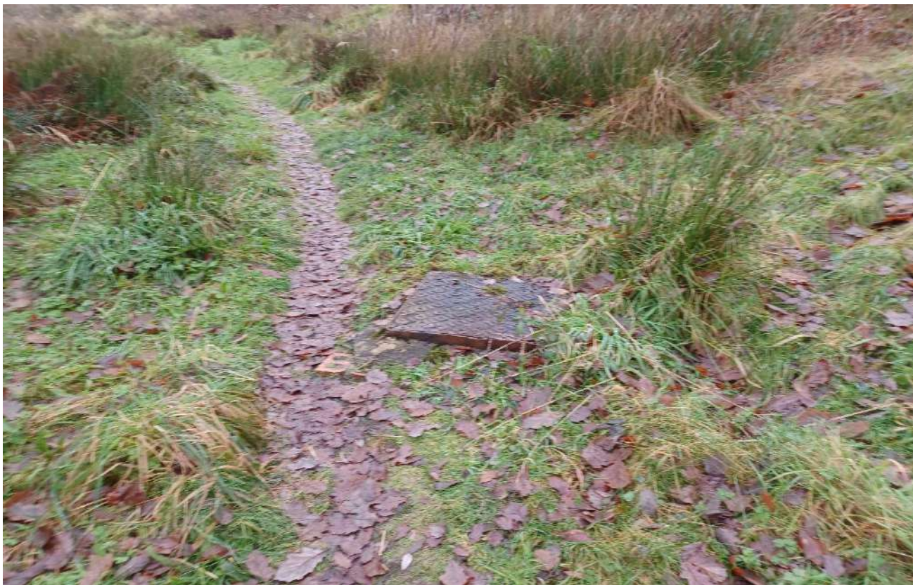
24 Manhole along footpath (facing NE)
