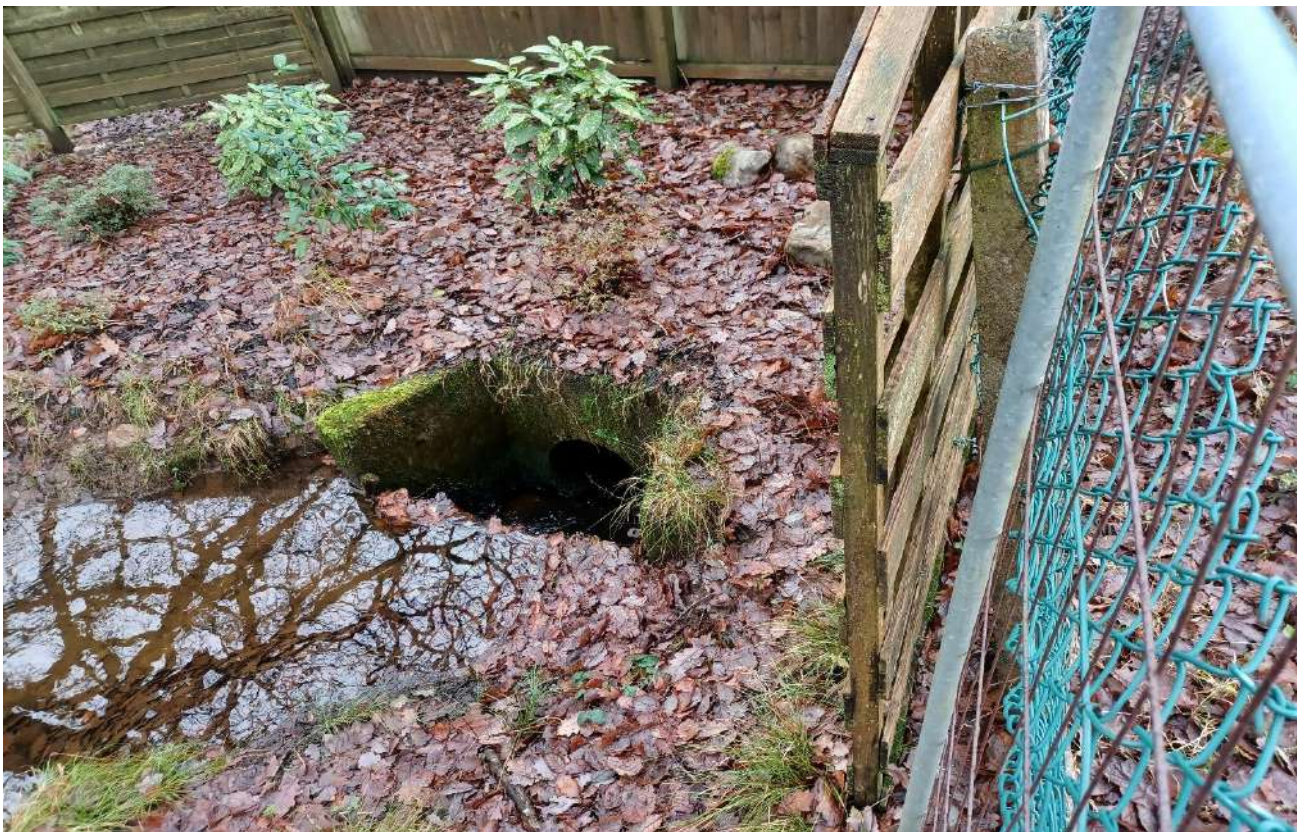
21 Offsite stream and drain - poss. beneath site
