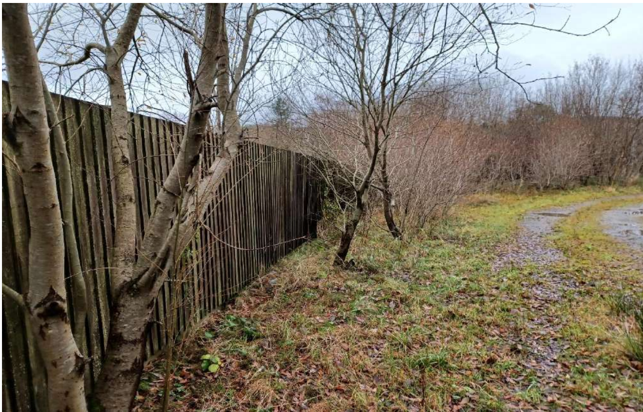
14 Site boundary (facing NW)
