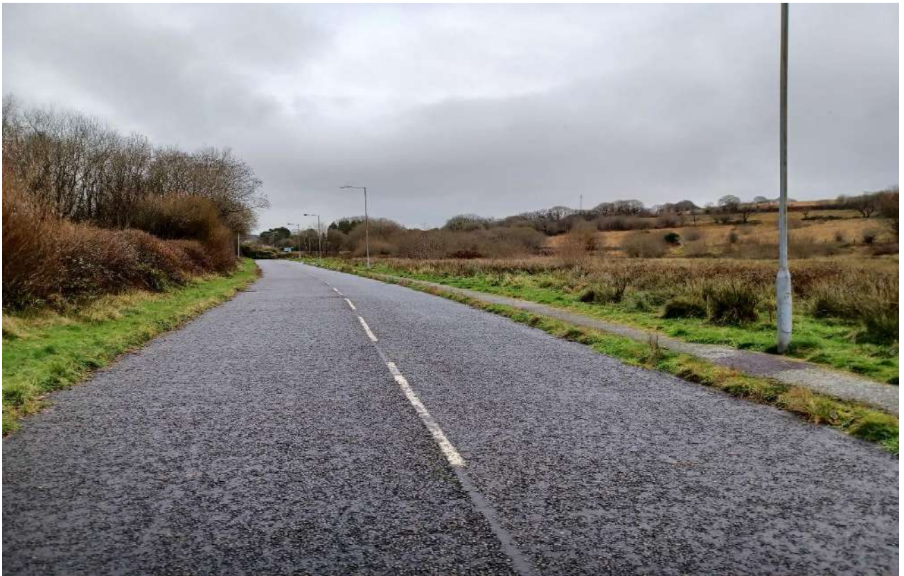
27 Blocked off road (facing NE)
