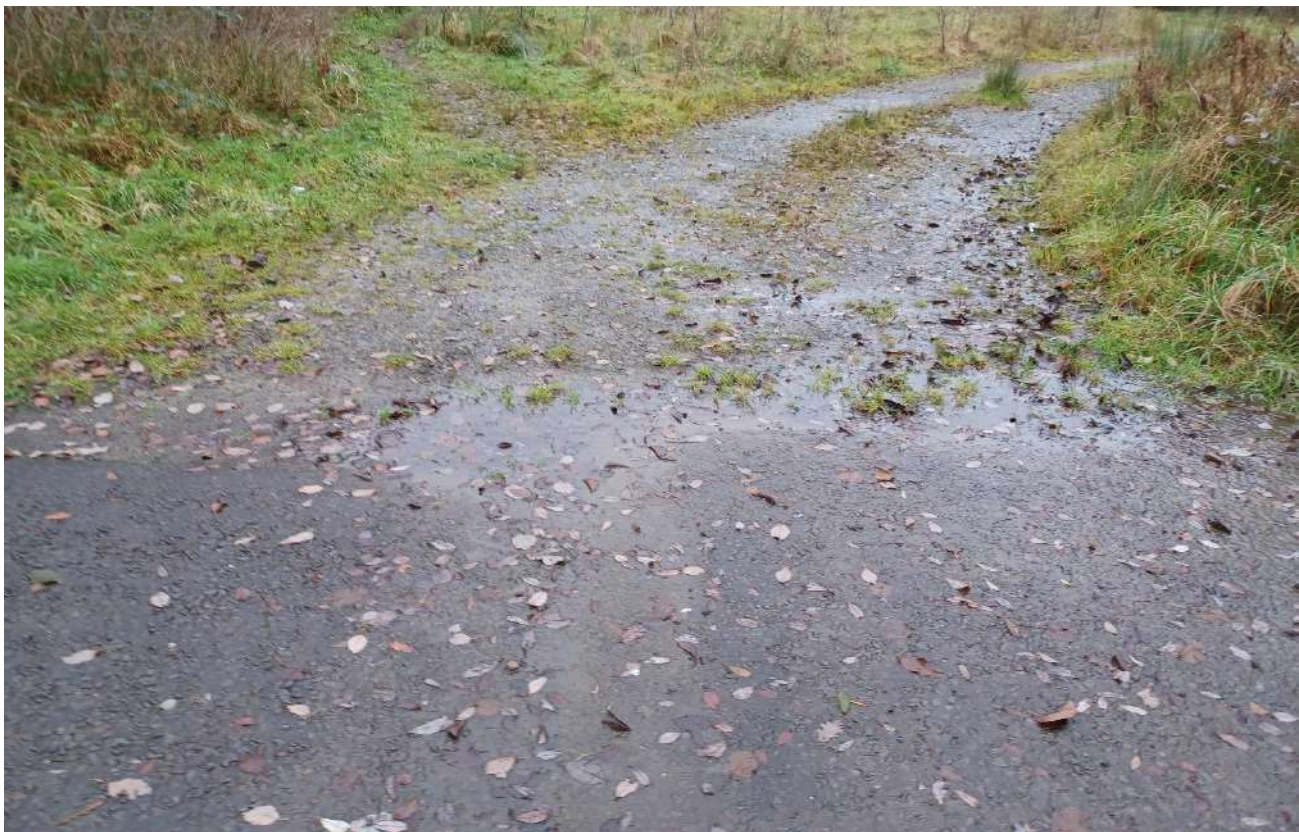
6 Track through site (facing SE)
