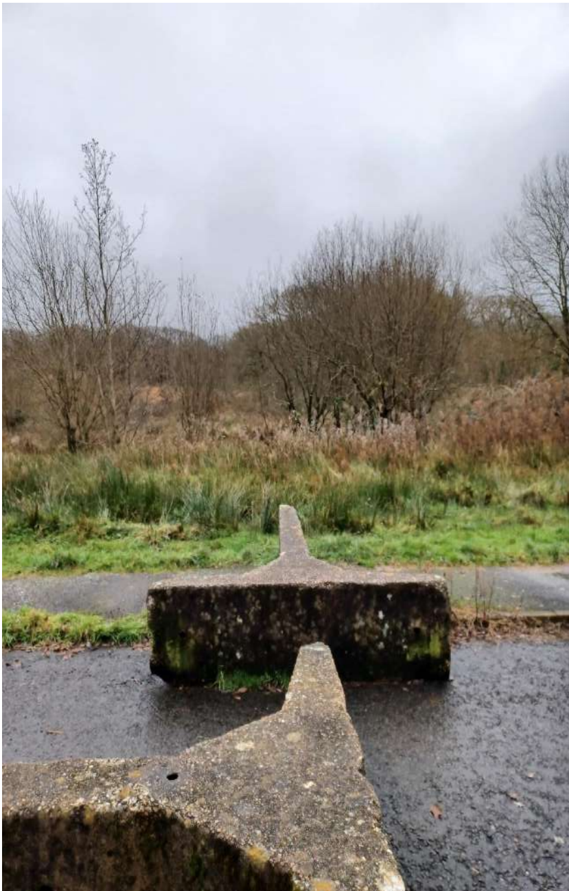
31 Block obstructions in road and site (facing SE)
