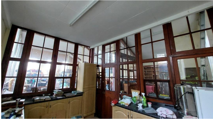
Photo Ref 94: Internal view of the Kitchen ceiling, wall panels and door.
