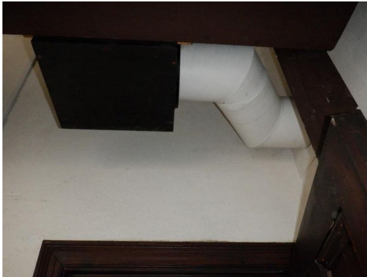
Photo Ref 116: View of ducting in room 3.
