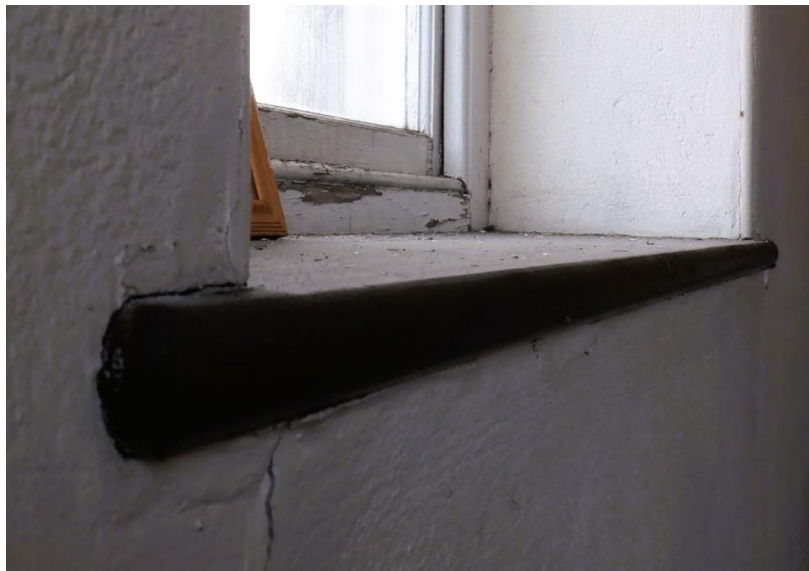
Photo Ref 105: Detail of the second floor window sill, this detail is the same for all the windows in room 1 to room 7.
