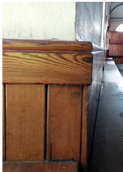
Photo Ref 149: Detail of first floor timber lower part of the window arch.
