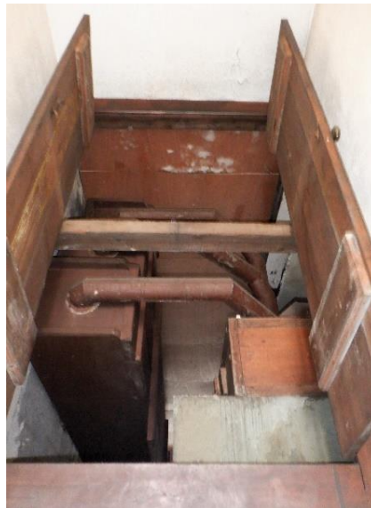
Photo Ref 127: View of the access door to the closet showing the organ machinery.
