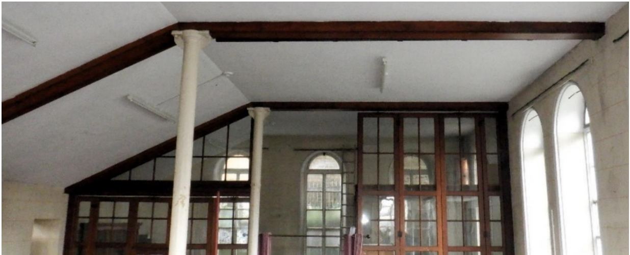
Photo Ref 87: Detail of the hall screen, ceiling and columns.
