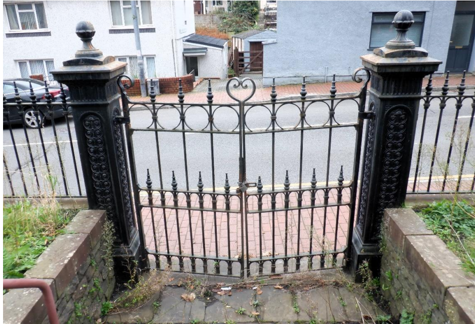
Photo Ref 170: View of the gates from the chapel main entrance towards the A4230.
