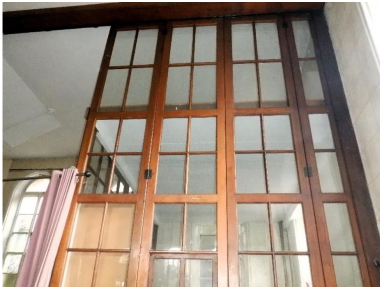
Photo Ref 89: Wood and glass full height, articulated panel that separates the hall area from the kitchen and side entrance. View from hall towards the kitchen.
