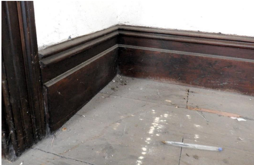
Photo Ref 106: Close-up of the skirting board on room 1, this detail is the same for all the skirting boards in room 1 to room 7.
