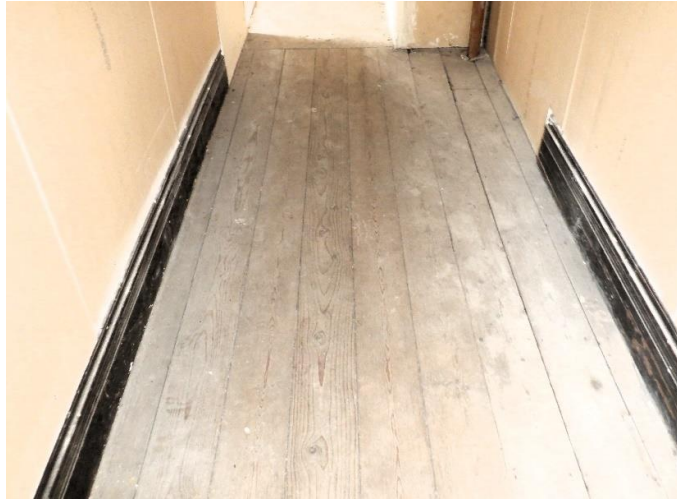
Photo Ref 104: Existing floor to the first floor in the back area of the chapel. View from staircase access.
