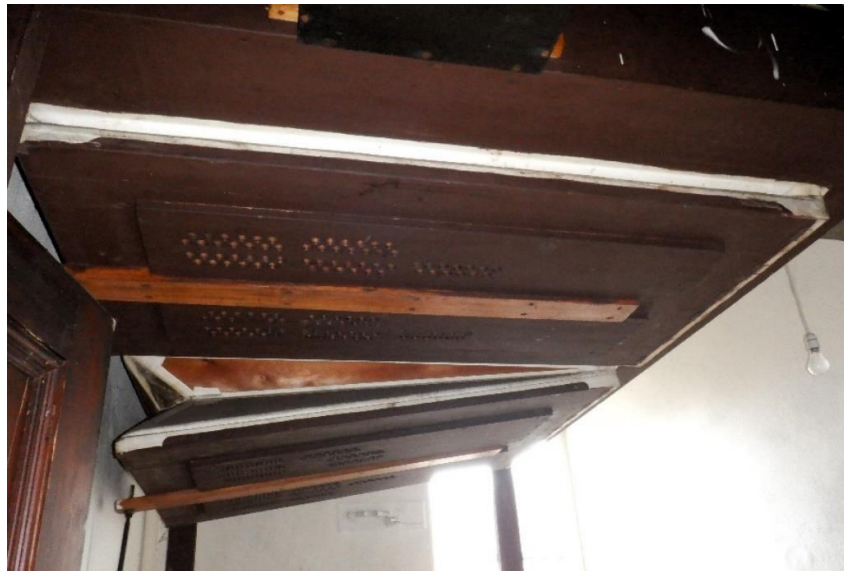
Photo Ref 113: Close-up view of the upper part of the bellows.
