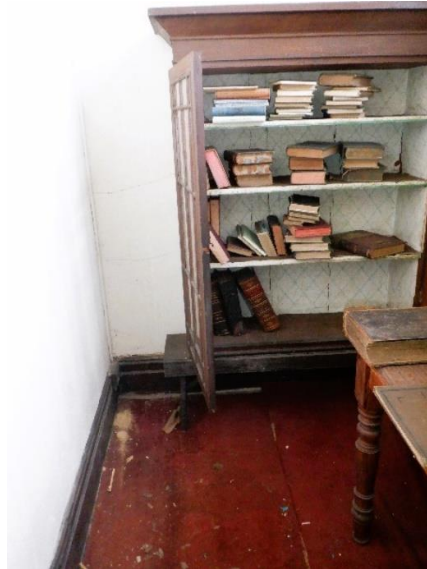
Photo Ref 124: Overall view of room 6.
