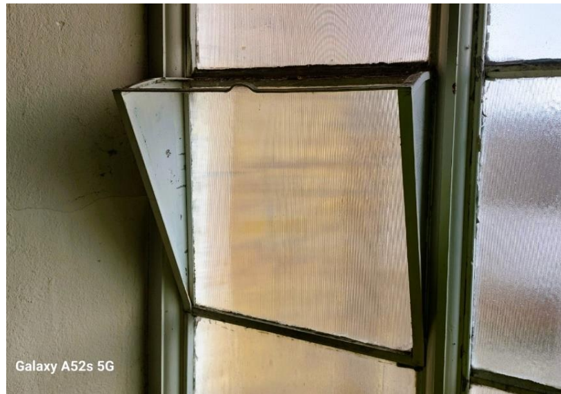
Photo Ref 148: Close-up window opener.
