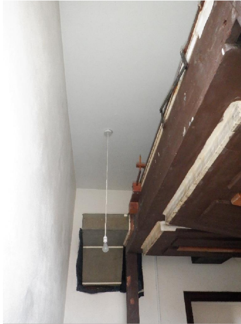
Photo Ref 118: Overall view of the upper part of the bellows.
