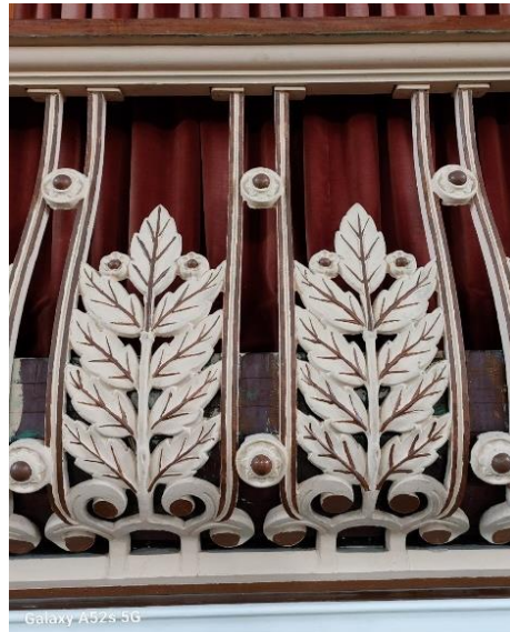
Photo Ref 140: Exterior view of the decorative detail of the metal railing with wooden handrails surrounding the Gallery.
