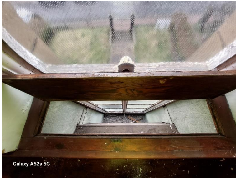
Photo Ref 158: Close-up view of the vent flap (open) showing the full length of the window.
