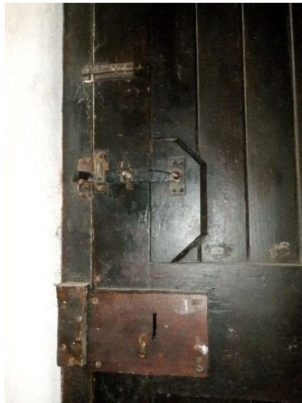
Photo Ref 99: Close-up view of the door locks detail.
