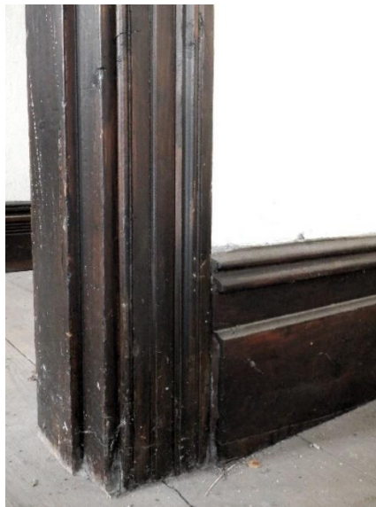
Photo Ref 107: Close-up view of the skirting board and architrave to room 1, this detail is the same for all the skirting boards and door frames in room 1 to room 7.
