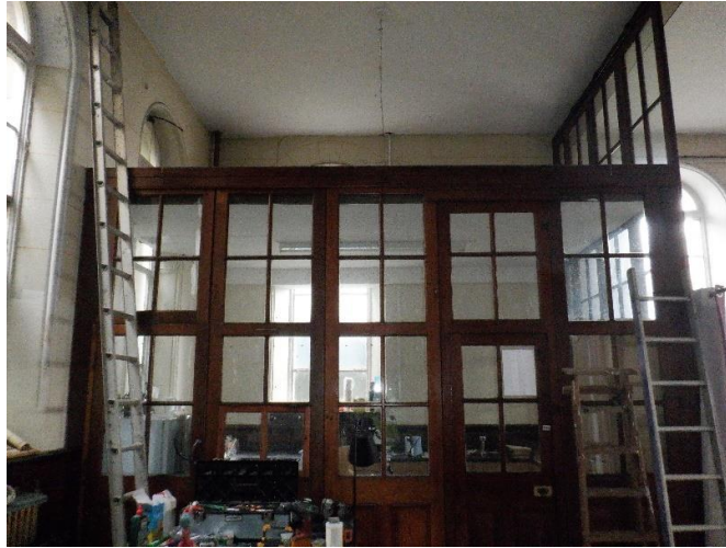
Photo Ref 92: Front view of the Kitchen panels and door.
