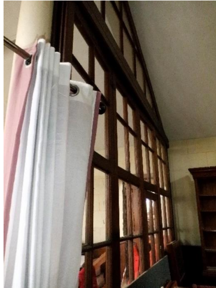
Photo Ref 96: Wood and glass full height, articulated panel that separates the hall area from the kitchen and side entrance. View from Kitchen towards the hall.
