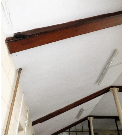
Photo Ref 86: Detail of the inclined part of the hall ceiling, this area is underneath organ.
