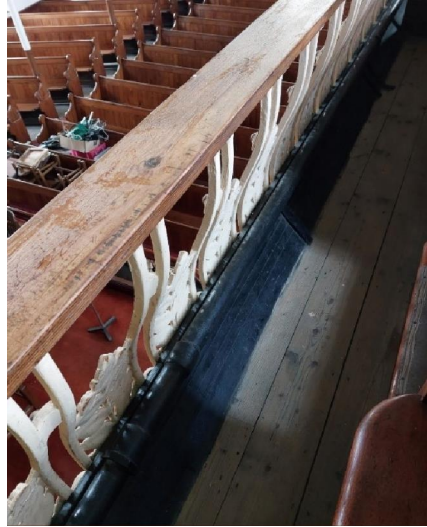
Photo Ref 142: Top view of the metal railing that surrounds the gallery.
