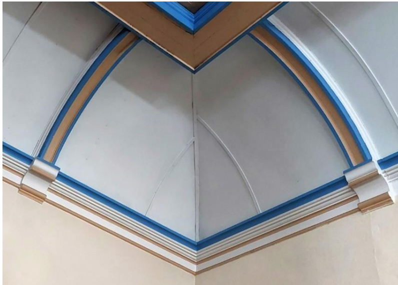
Photo Ref 162: Close-up view of the ceiling corner detail.
