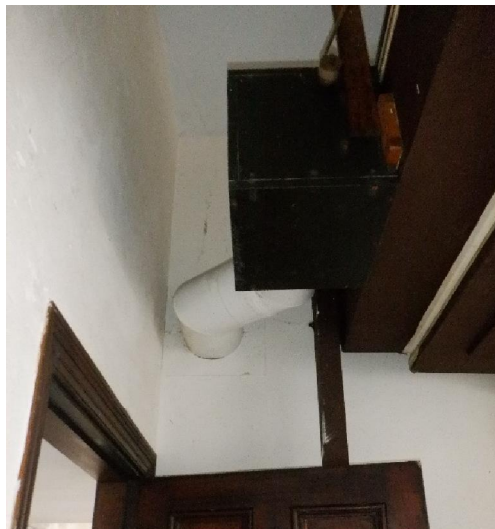
Photo Ref 117: View of ducting in room 3.
