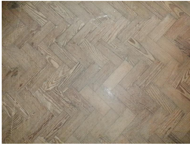
Photo Ref 90: Existing floor finish to the Hall.
