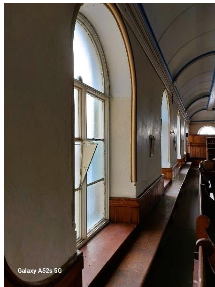
Photo Ref 147: View of the first-floor windows in the Gallery.
