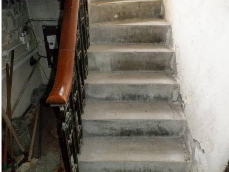
Photo Ref 100: Front view of the access staircase to the first floor from the West elevation.
