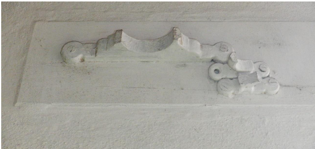
Photo Ref 119: Decorative timber to the left side of the window in room 3.
