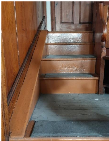
Photo Ref 131: Stairs that connect the gallery of the chapel with the rear part of the Sunday School.
