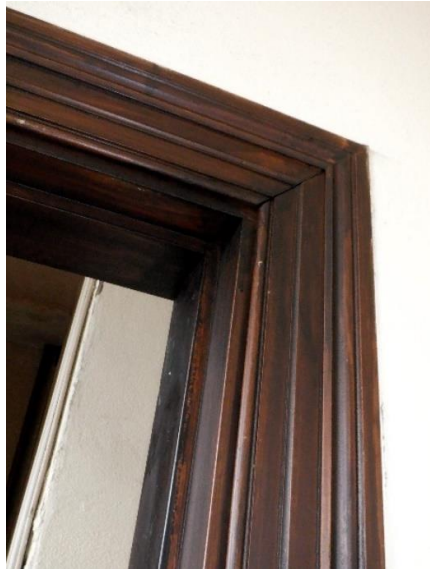
Photo Ref 108: Close-up view of the upper part of door frame/architrave from room 1, this detail is the same for all the door frames in room 1 to room 7.
