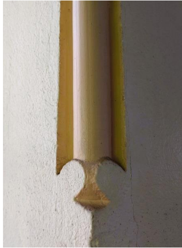
Photo Ref 150: Detail of decorative window arch. This is on all windows on the first floor.
