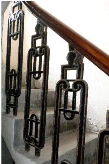
Photo Ref 101: Close-up view of the decorative steel balustrade, timber handrail.
