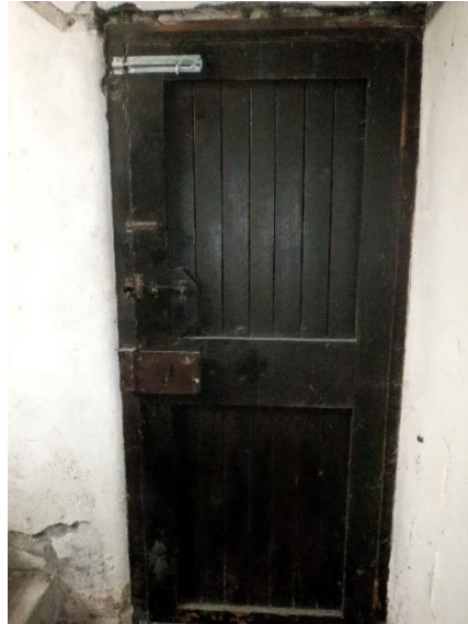
Photo Ref 98: Internal view of the west elevation exterior door.
