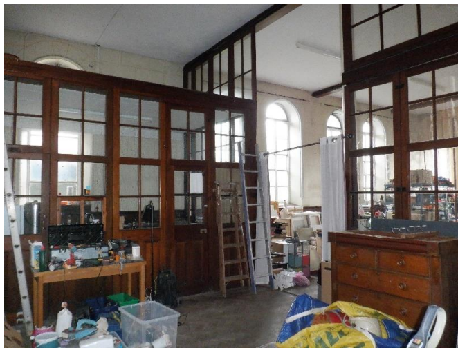
Photo Ref 91: Wood and glass full height, articulated panel that separates the Hall area from the kitchen and side entrance, the kitchen panel and the door to access the kitchen. View from side entrance towards the Kitchen.
