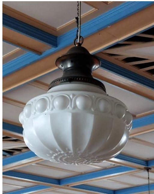
Photo Ref 167: Close-up view of one of the ceiling lamps, all the lamps in the ceiling are the same.
