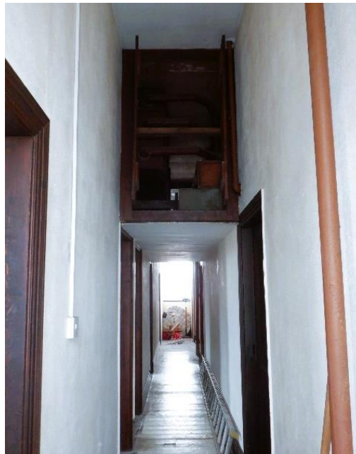
Photo Ref 125: General view of the first-floor hallway with the access door to the organ machinery open.
