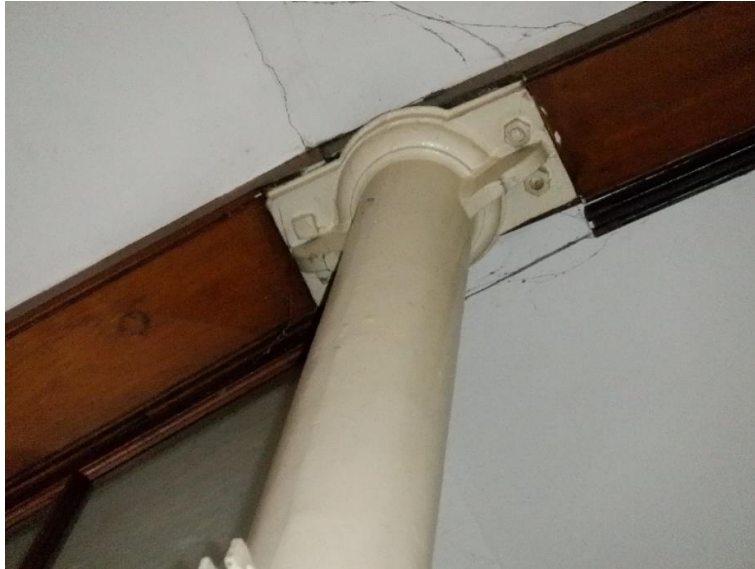
Photo Ref 88: Close-up view of the upper part of the hall column.
