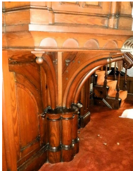
Photo Ref 81: Detail of the Gothic style mini column that supports the pulpit platform. Side view from the Altar.
