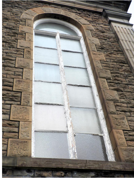
Photo Ref 13: Detail of side window of main facade. View from South elevation.
