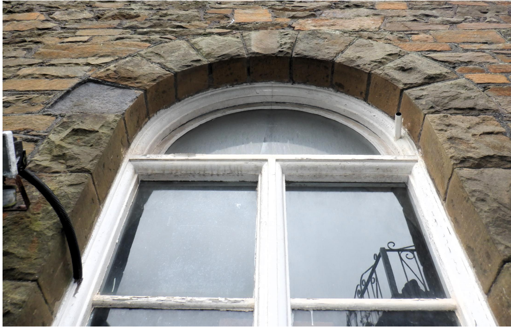
Photo Ref 29: Detail of the upper arch of one of the round headed windows at the back of the chapel. View from North elevation.
