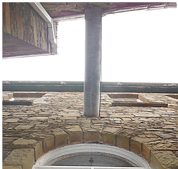
Photo Ref 36: Detail of the ventilation pipe from the organ of the chapel. View from West elevation.
