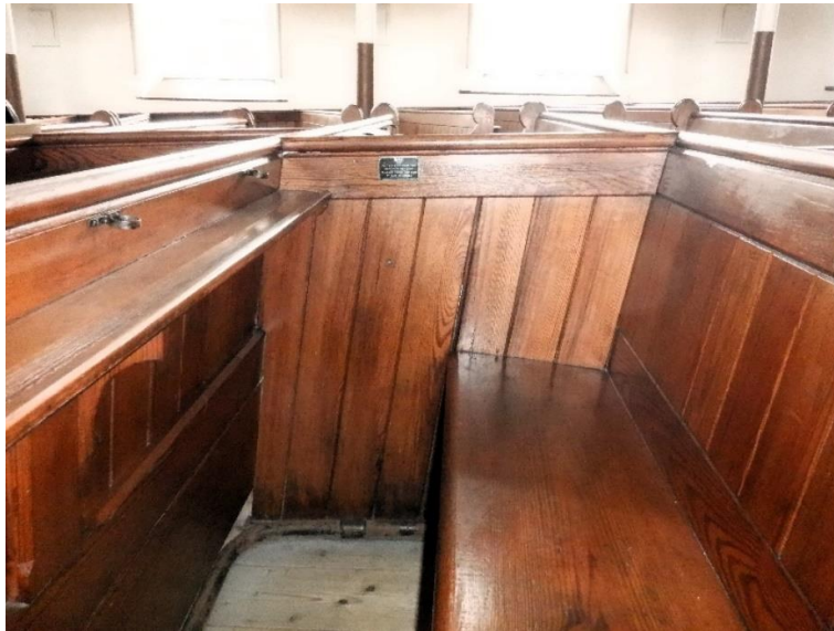
Photo Ref 66: View of the central pew showing where the aluminium plate is installed.
