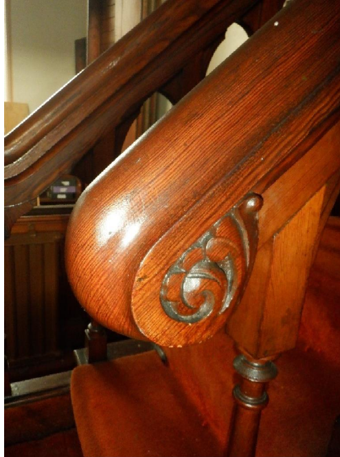
Photo Ref 74: Close-up view of the newel post to access the pulpit platform.
