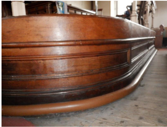
Photo Ref 70: Close-up view of the predella (altar platform) along with the heating pipe.
