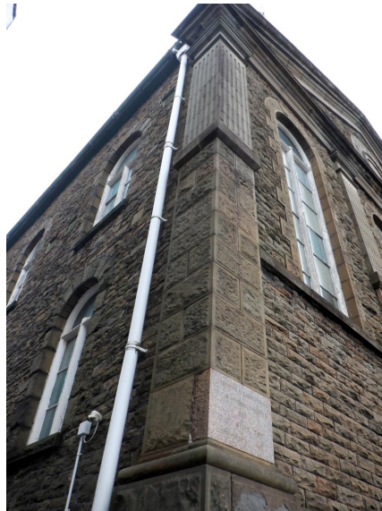
Photo Ref 16: Lateral pilaster detail. View from West elevation.
