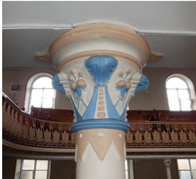
Photo Ref 61: Close-up view of the upper part of the column.
