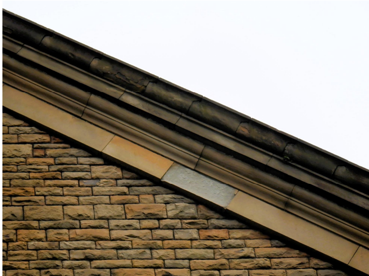
Photo Ref 05: Detail of the joint between the roof and front façade of the chapel showing the moulded cornice. View from South elevation.
