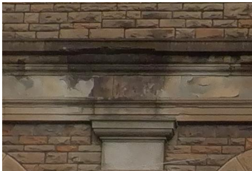
Photo Ref 10: Decorative Cornice and Pilaster detail on the top of the main façade of the chapel. View from South elevation.
