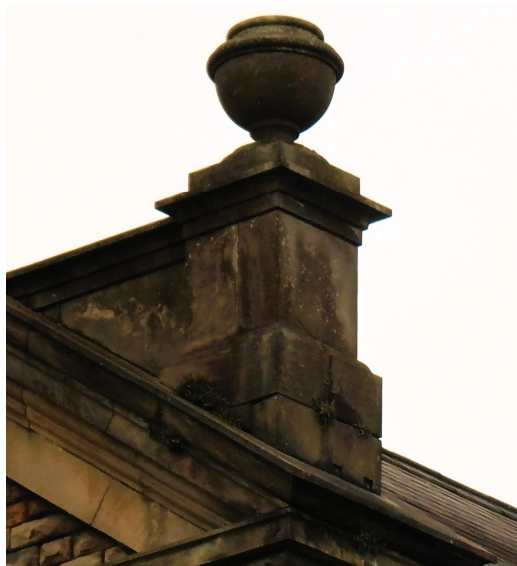
Photo Ref 08: Decorative detail (Urn) on the top lateral of the main façade of the chapel. View from East elevation.
