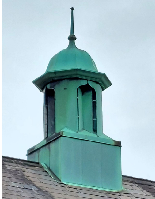
Photo Ref 23: Detail of the central cupola of the chapel's ventilation system. View from West elevation.
