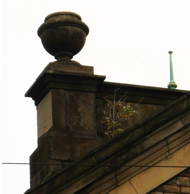
Photo Ref 09: Decorative detail (Urn) on the top lateral of the main façade of the chapel. View from South elevation.
