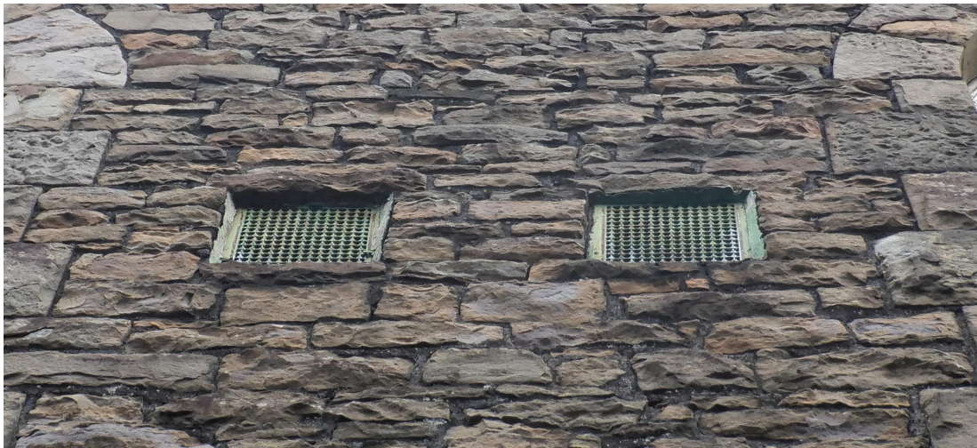
Photo Ref 32: Double grille detail of the ventilation system. View from West elevation.
