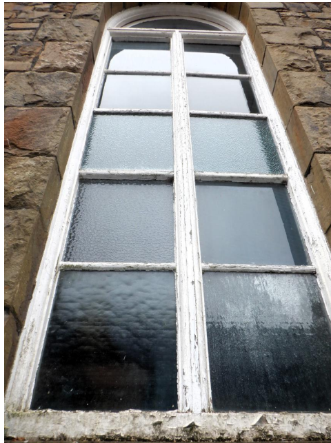
Photo Ref 28: Detail of one of the ground-floor round headed side windows of the chapel. View from East elevation.
