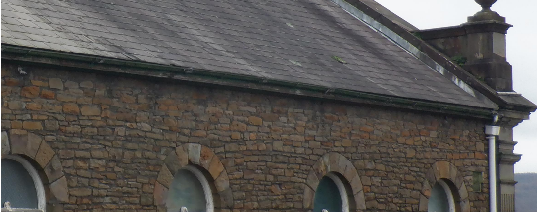
Photo Ref 39: Detail of the joint between the roof and lateral façade of the chapel. View from West elevation.
