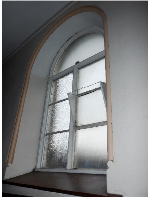
Photo Ref 55: Internal view of a ground floor, bottom hung window with stay. All ground floor windows have the same detail.
