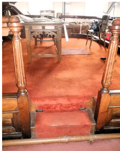
Photo Ref 71: Internal view of the predella along the access steps and the table of the altar. View from the left aisle towards the altar.
