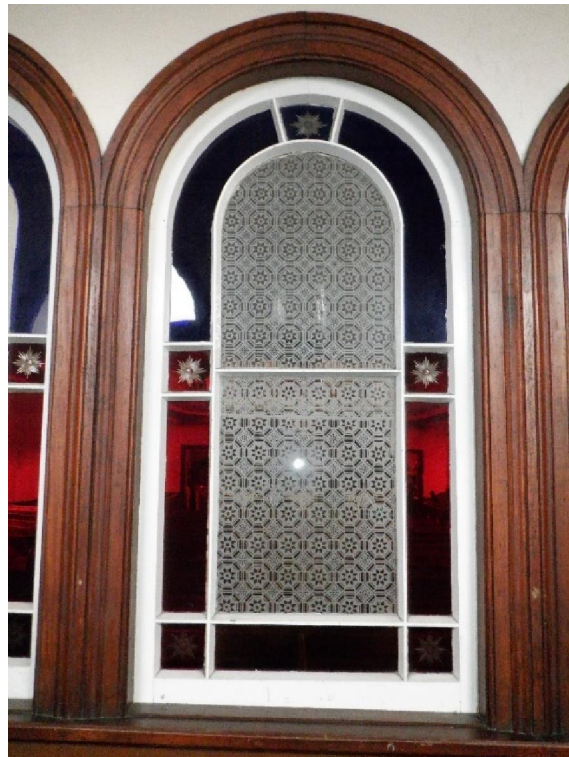
Photo Ref 45: Close-up view of one of the triplet of semi-circular arch windows.
