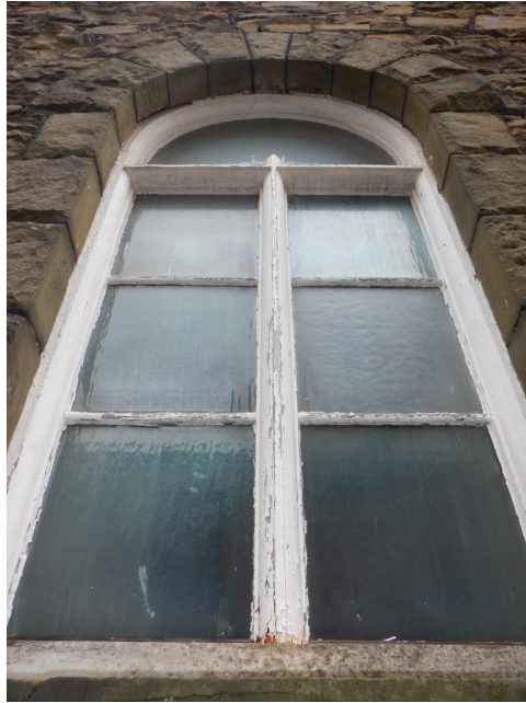
Photo Ref 33: Detail of one of the ground-floor round headed side windows of the chapel. View from West elevation.
