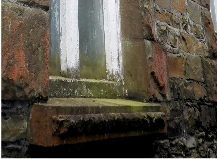
Photo Ref 31: Detail of the semi dressed rustic window sill of one of the windows at the back of the chapel. View from North elevation.
