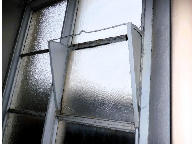
Photo Ref 56: Internal view of window opening, all ground floor windows have the same detail.
