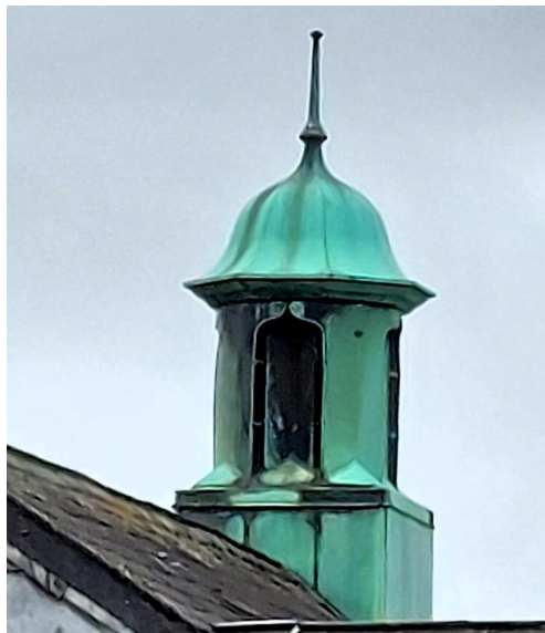
Photo Ref 22: Detail of the central cupola of the chapel's ventilation system. View from North elevation.
