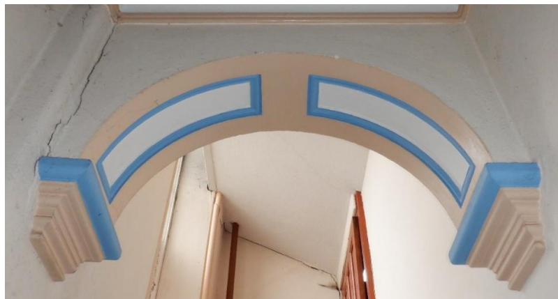
Photo Ref 41: Arch with painted moulded decoration, this arch is located at the entrance to the stairs leading to the first floor of the chapel. Front view from the Lobby.
