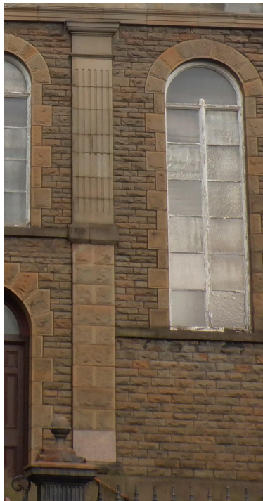
Photo Ref 12: Front fluted pilaster detail. View from South elevation.
