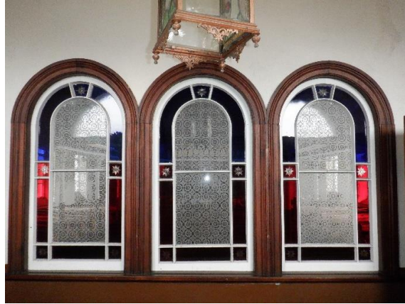
Photo Ref 44: Triplet of semi-circular arch windows composed of decorative stained-glass located on the wall that separates the Lobby from the Chapel. Front view from the main entrance.
