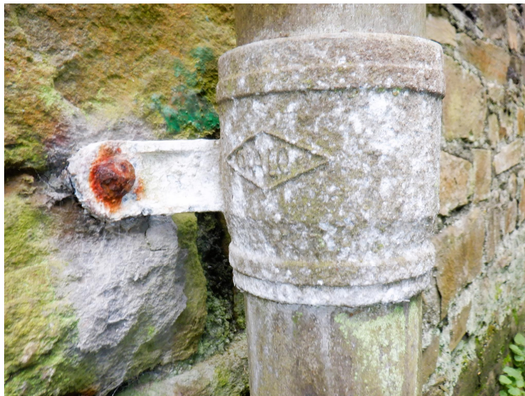
Photo Ref 30: Detail of the clip that connects the drain pipe to the wall. View from the North elevation.
