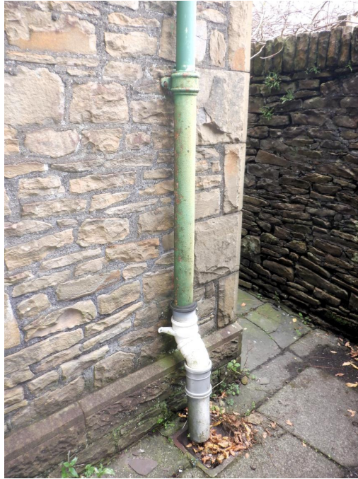
Photo Ref 19: Detail of the lower part of the drain pipe. View from South elevation.
