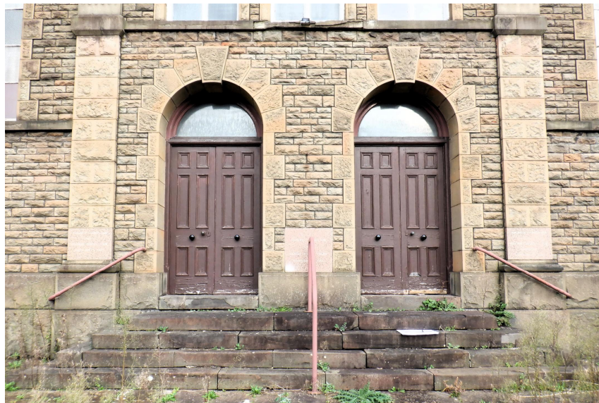
Photo Ref 14: Detail of the main painted panelled doors with arched fanlights of the chapel. View from South elevation.
