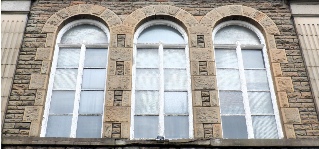
Photo Ref 11: Trio of round headed windows on the front façade. View from South elevation.
