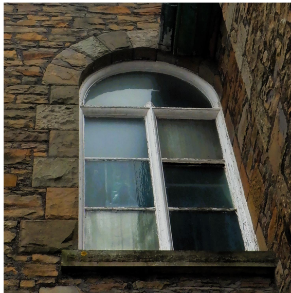
Photo Ref 24: Detail of one of the first-floor round headed side windows of the chapel. View from East elevation.
