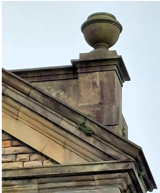
Photo Ref 07: Decorative detail (Urn) on the top lateral of the main façade of the chapel. View from South elevation.
