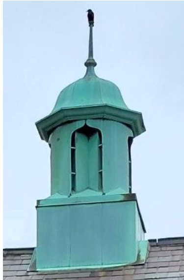
Photo Ref 21: Detail of the central cupola of the chapel's ventilation system. View from East elevation.
