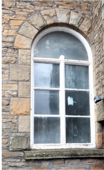
Photo Ref 25: Detail of one of the ground-floor round headed side windows of the chapel. View from East elevation.
