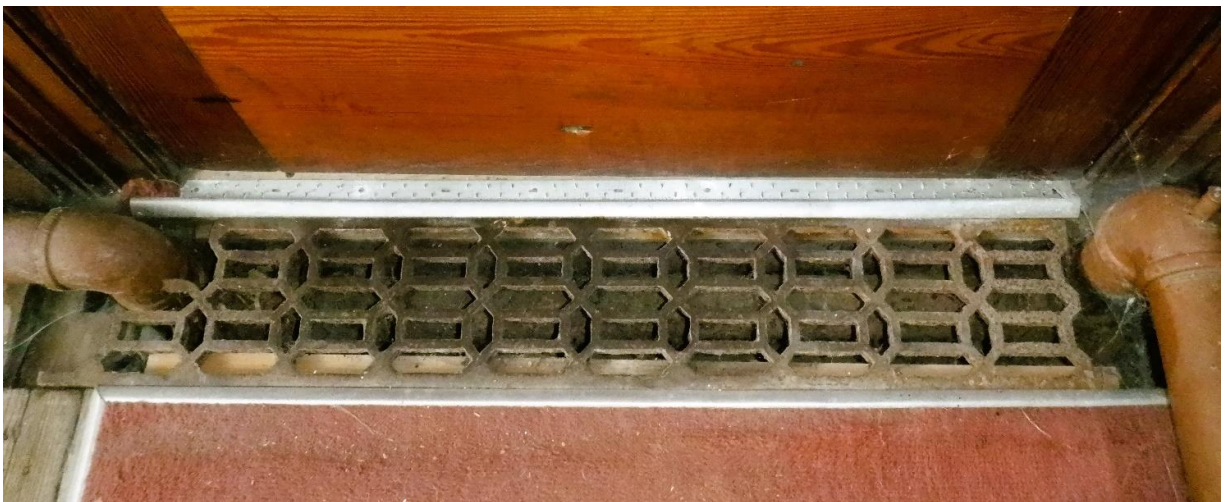
Photo Ref 85: Close-up view of the grille detail.
