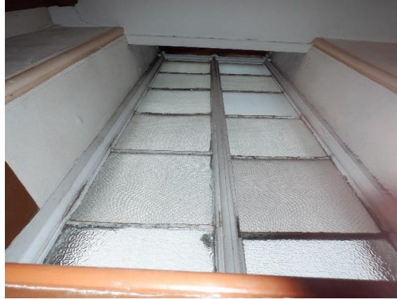
Photo Ref 46: Internal view of one of the side windows of the front facade. View from the access stairs to the first floor upwards.
