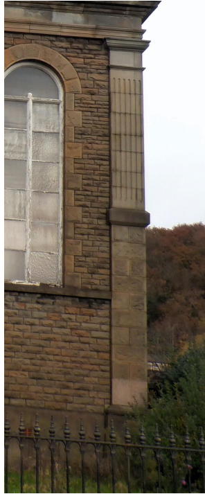
Photo Ref 15: Lateral fluted pilaster detail. View from South elevation.
