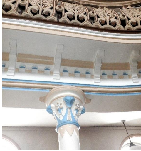
Photo Ref 60: Upper part of the column seen from the nave.
