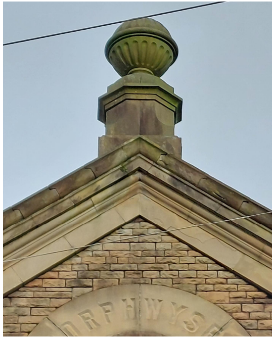
Photo Ref 01: Decorative Finial detail on the top centre of the main façade of the chapel with moulded cornice. View from South elevation.
