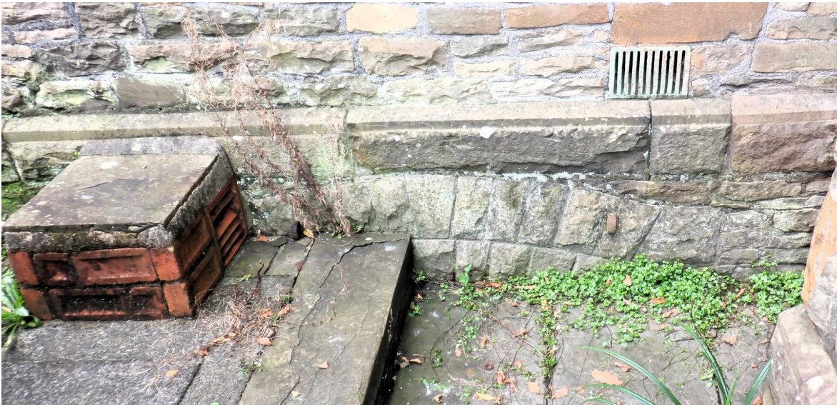
Photo Ref 26: Detail of the interior door arch of the basement. View from East elevation.
