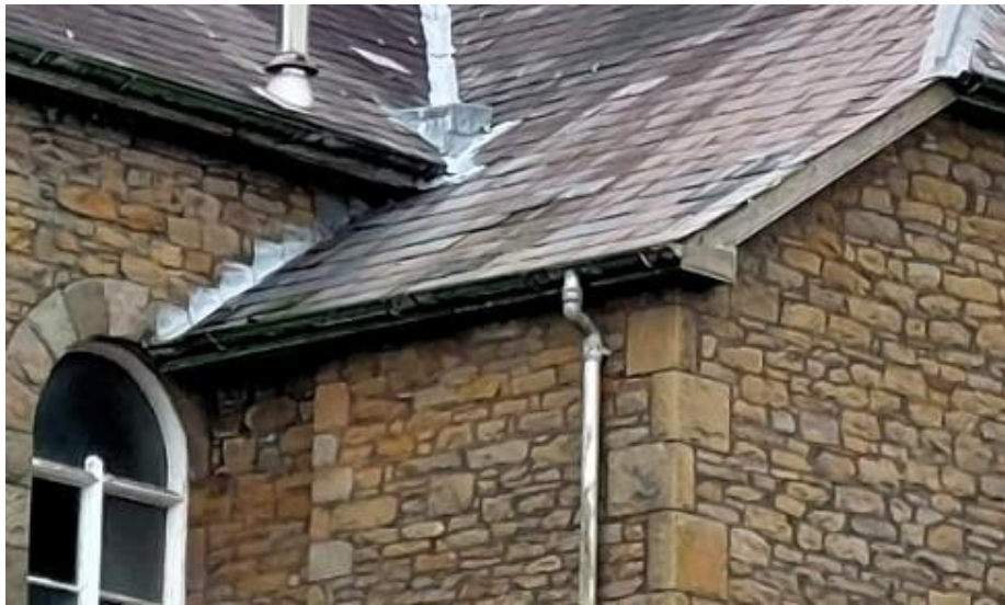
Photo Ref 20: Detail of the top part of the drain pipe and roof. View from East elevation.
