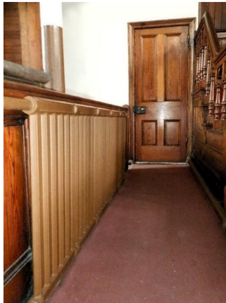
Photo Ref 83: View to the hall access door, along one of the many radiators of the chapel.
