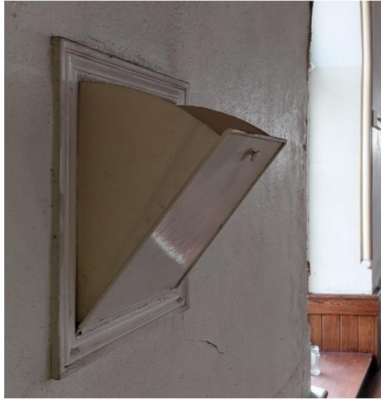
Photo Ref 54: Open metal ventilation shutter.
