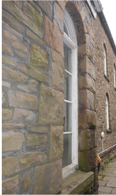
Photo Ref 35: Detail of one of the round headed ground-floor side windows of the chapel. View from West elevation.
