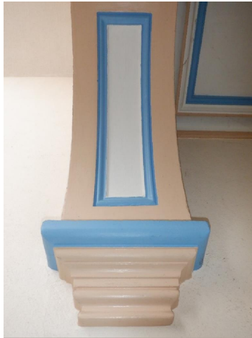
Photo Ref 42: Arch with moulded decoration, this arch is located at the entrance to the stairs leading to the first floor of the chapel. Side view from the lobby.
