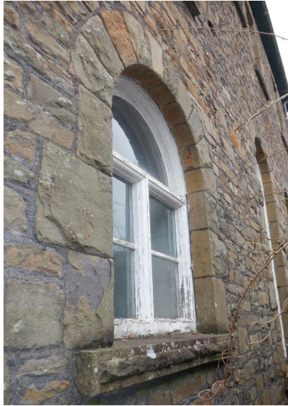
Photo Ref 27: Detail of the round headed staircase window. View from East elevation.
