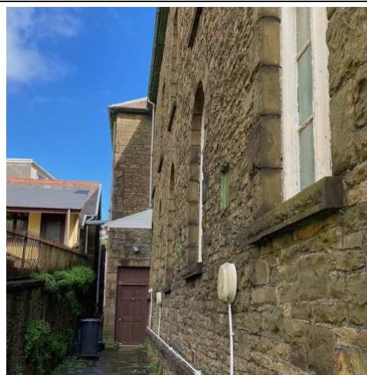
Figure 15. Lean-to porch on western elevation.
