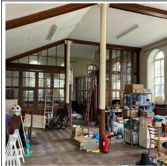
Figure 20. Ground floor of schoolroom (west).
