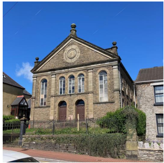
Figure 9. Front gable of the chapel, showing windows and doors.
