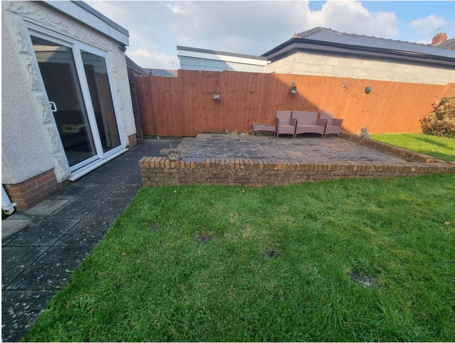
View of existing rear extension to be demolished and neighbours timber fence boundary and patio area.
