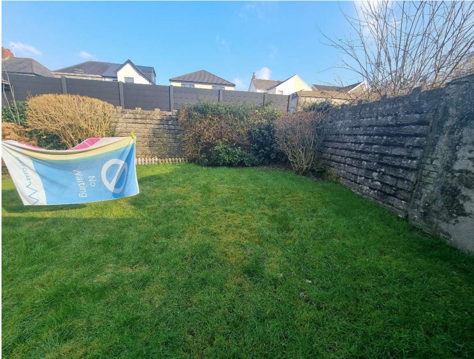
Rear lawn area with blockwork boundary walls to side and rear. These will remain unaltered.
