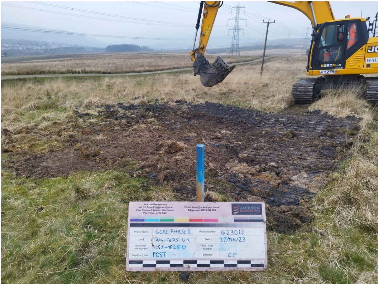
S2-TP280 Post Excavation
