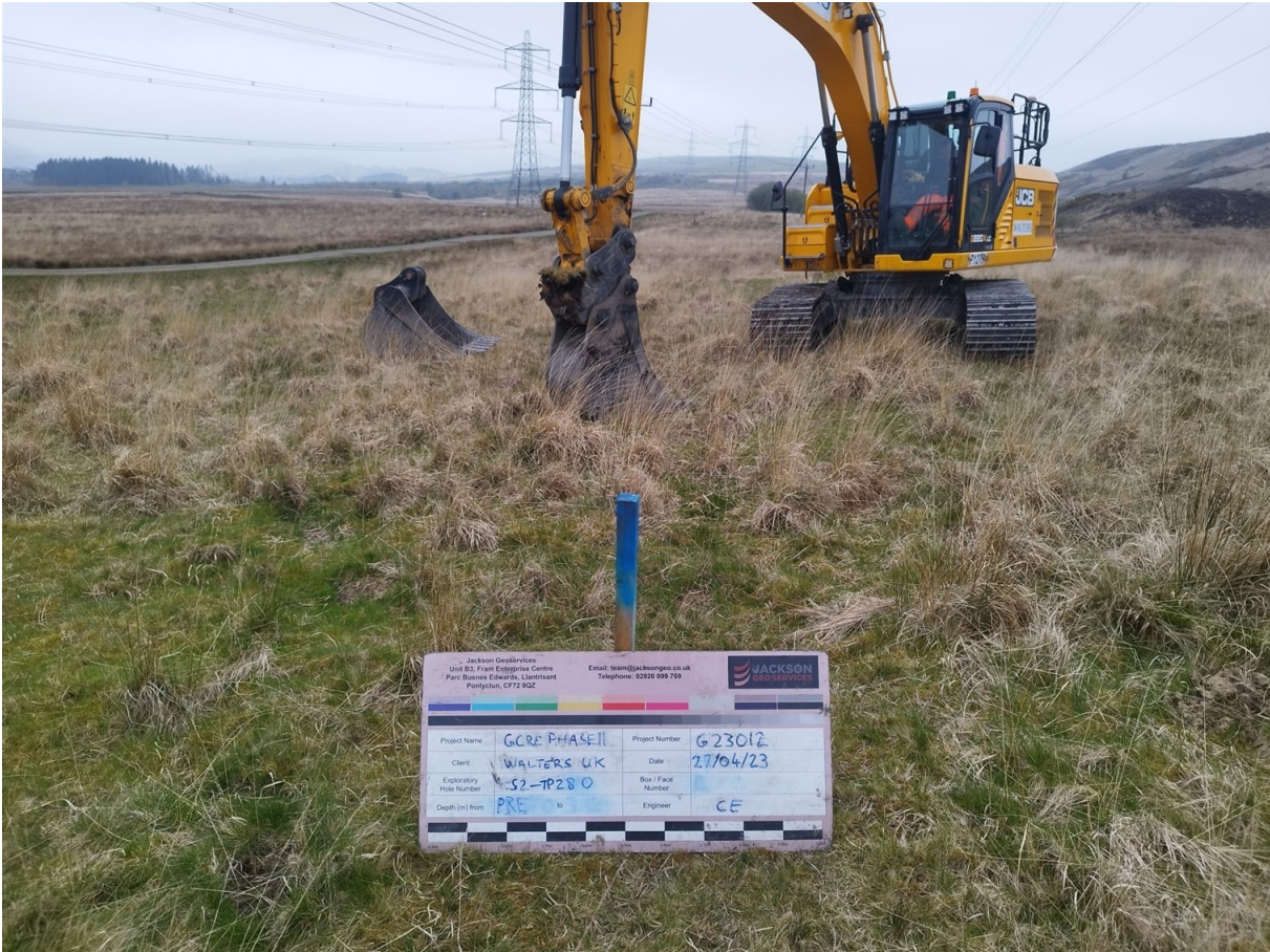
S2-TP280 Pre Excavation
