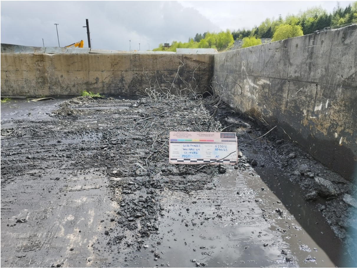
S2-TP284 Post Excavation
