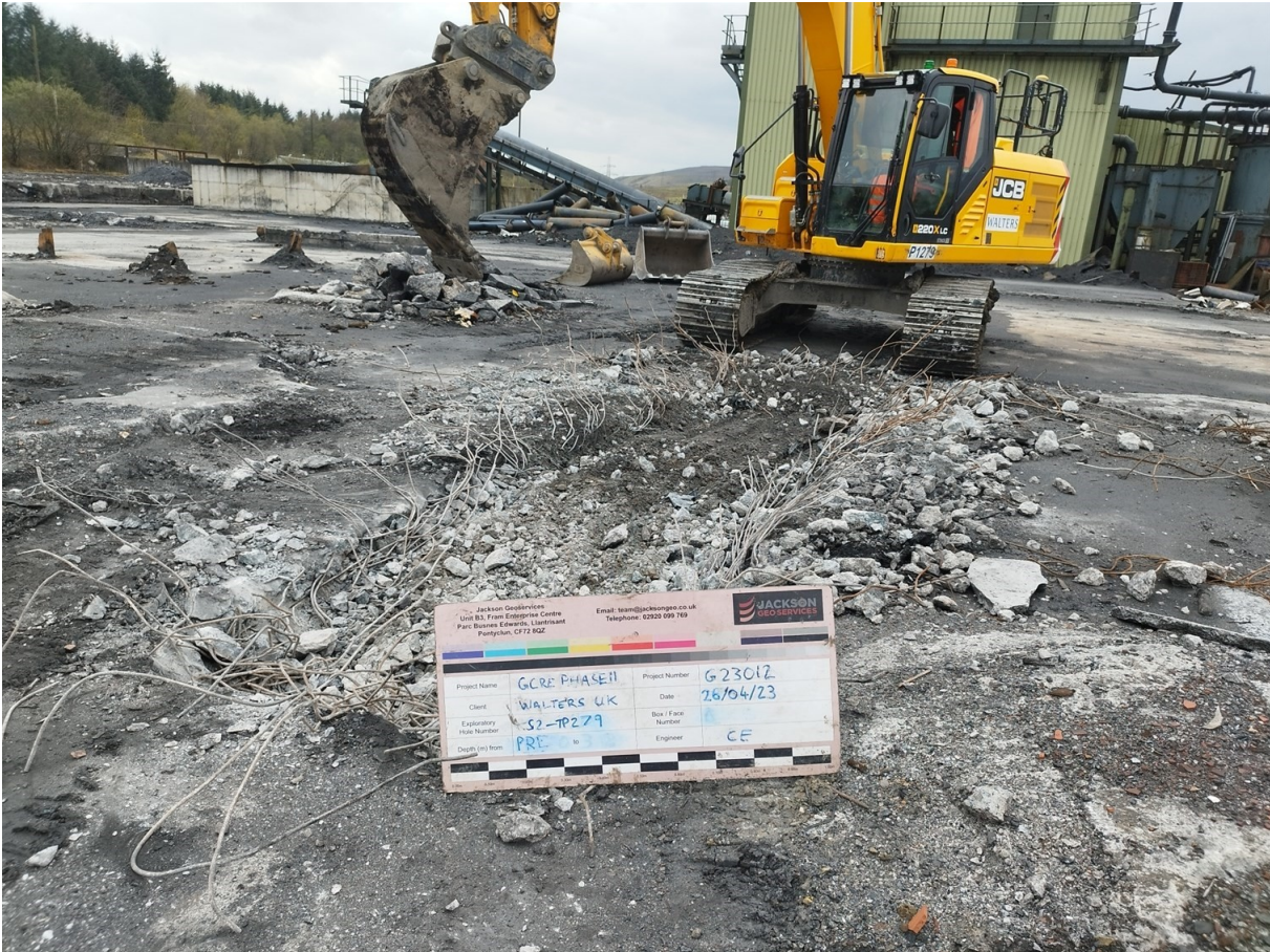
S2-TP279 Pre Excavation
