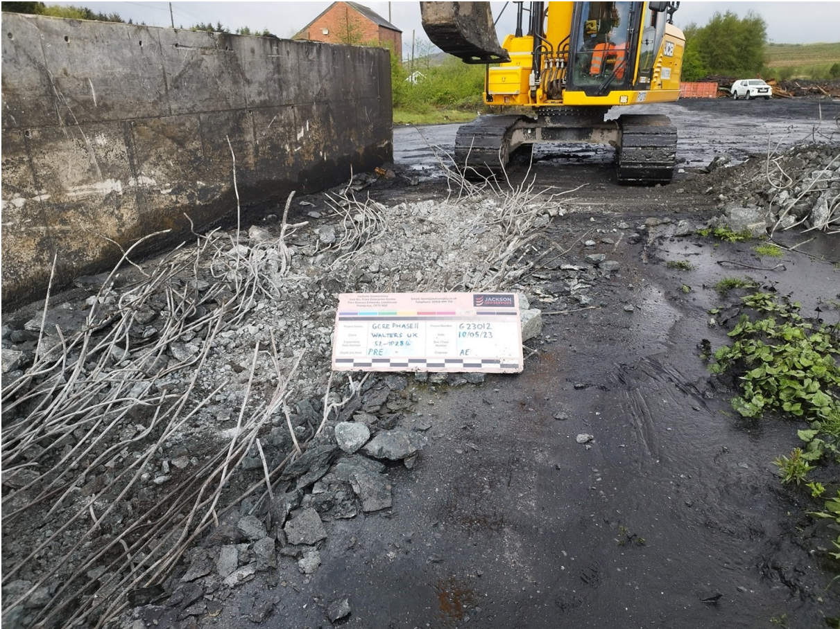
S2-TP284 Pre Excavation
