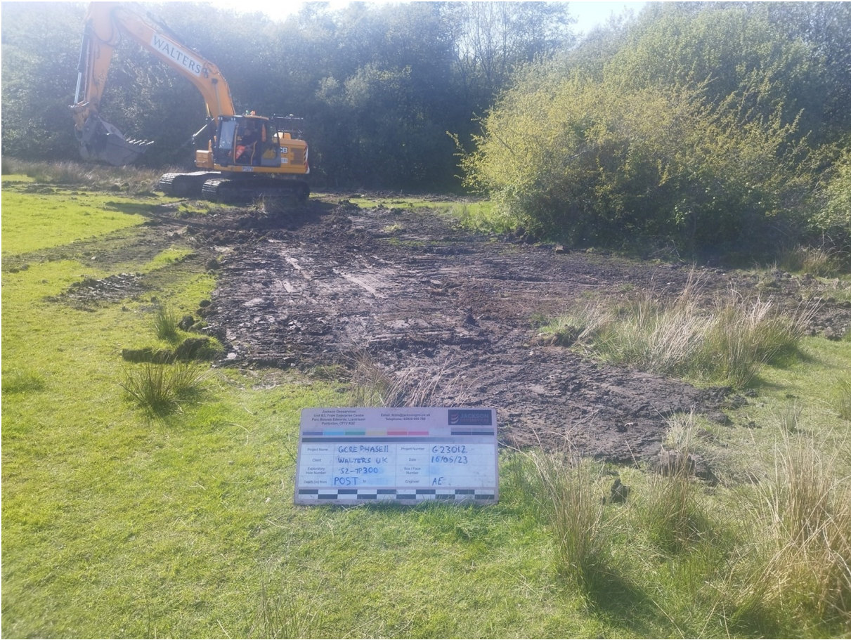
S2-TP300 Post Excavation
