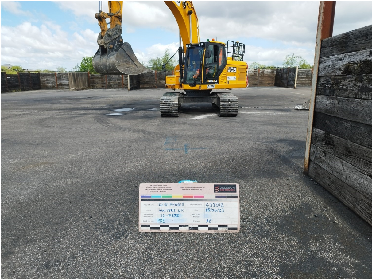
S2-TP272 Pre Excavation
