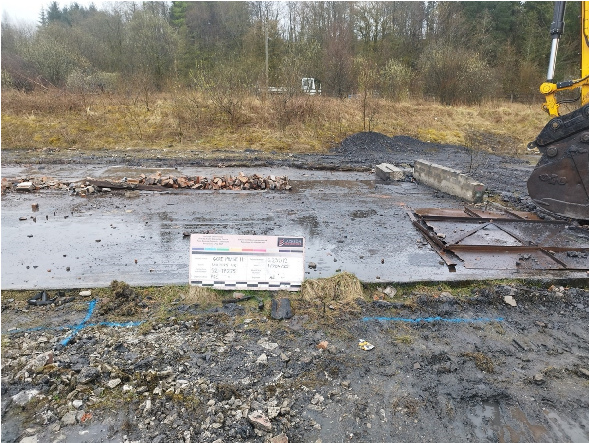
S2-TP275 Pre Excavation
