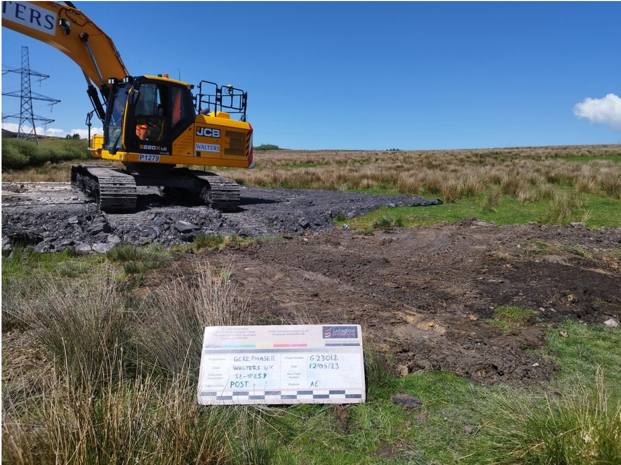
S2-TP259 Post Excavation
