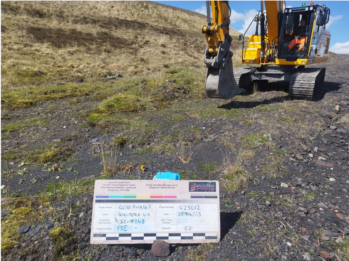
S2-TP243 Pre Excavation
