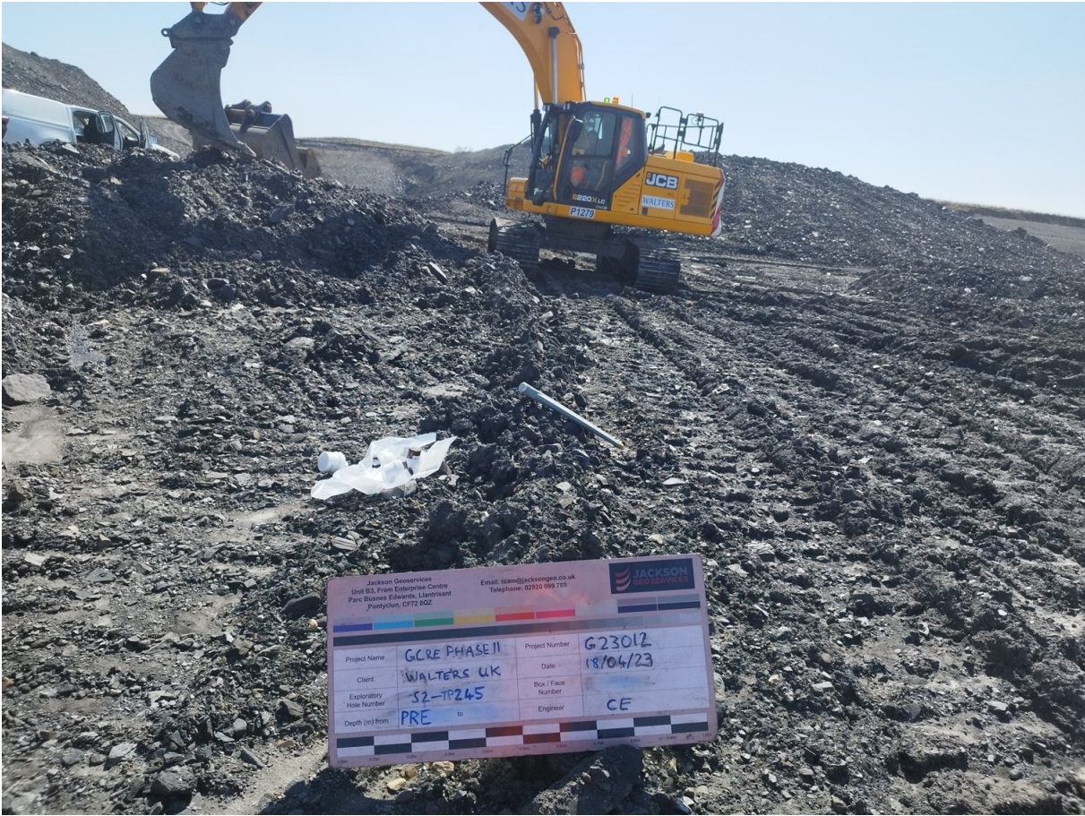
S2-TP245 Pre Excavation
