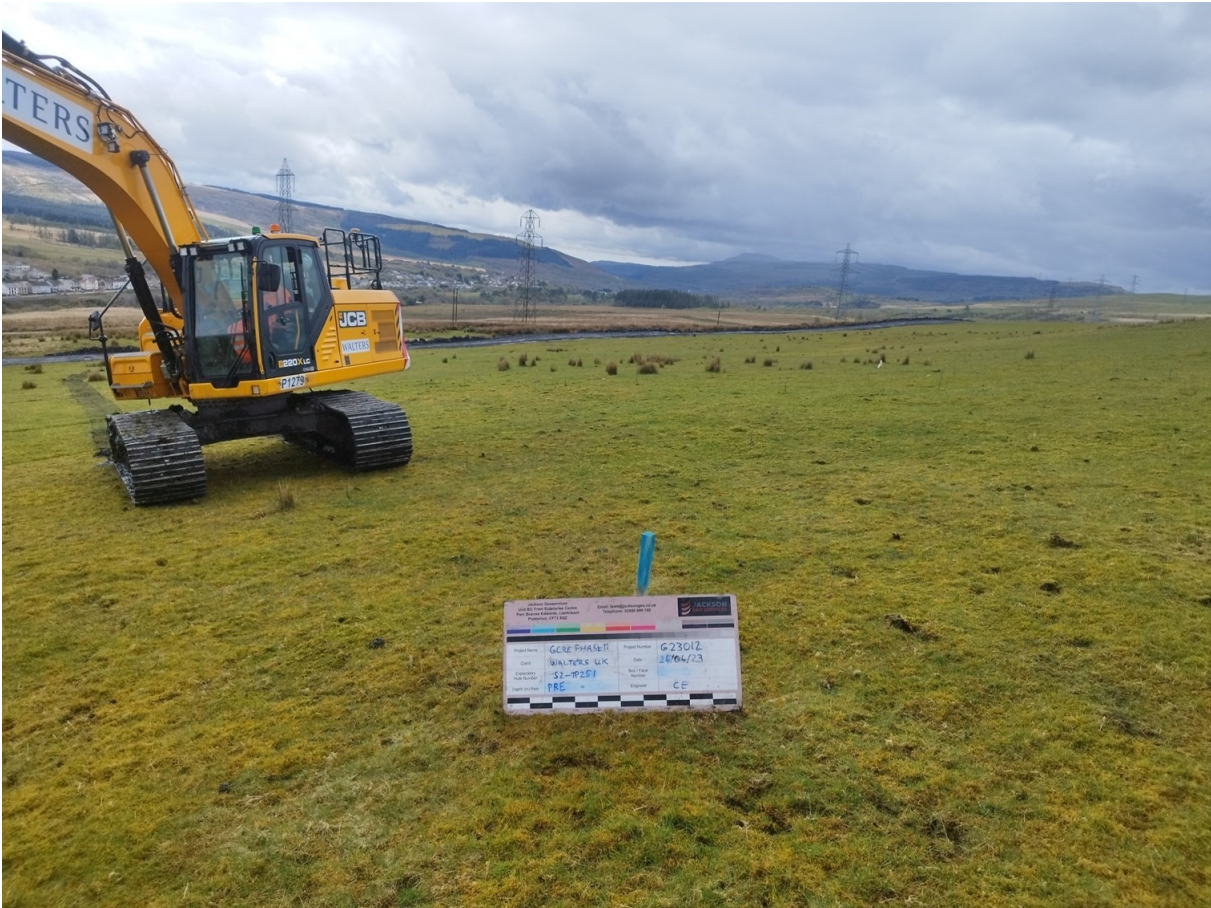
S2-TP252 Pre Excavation
