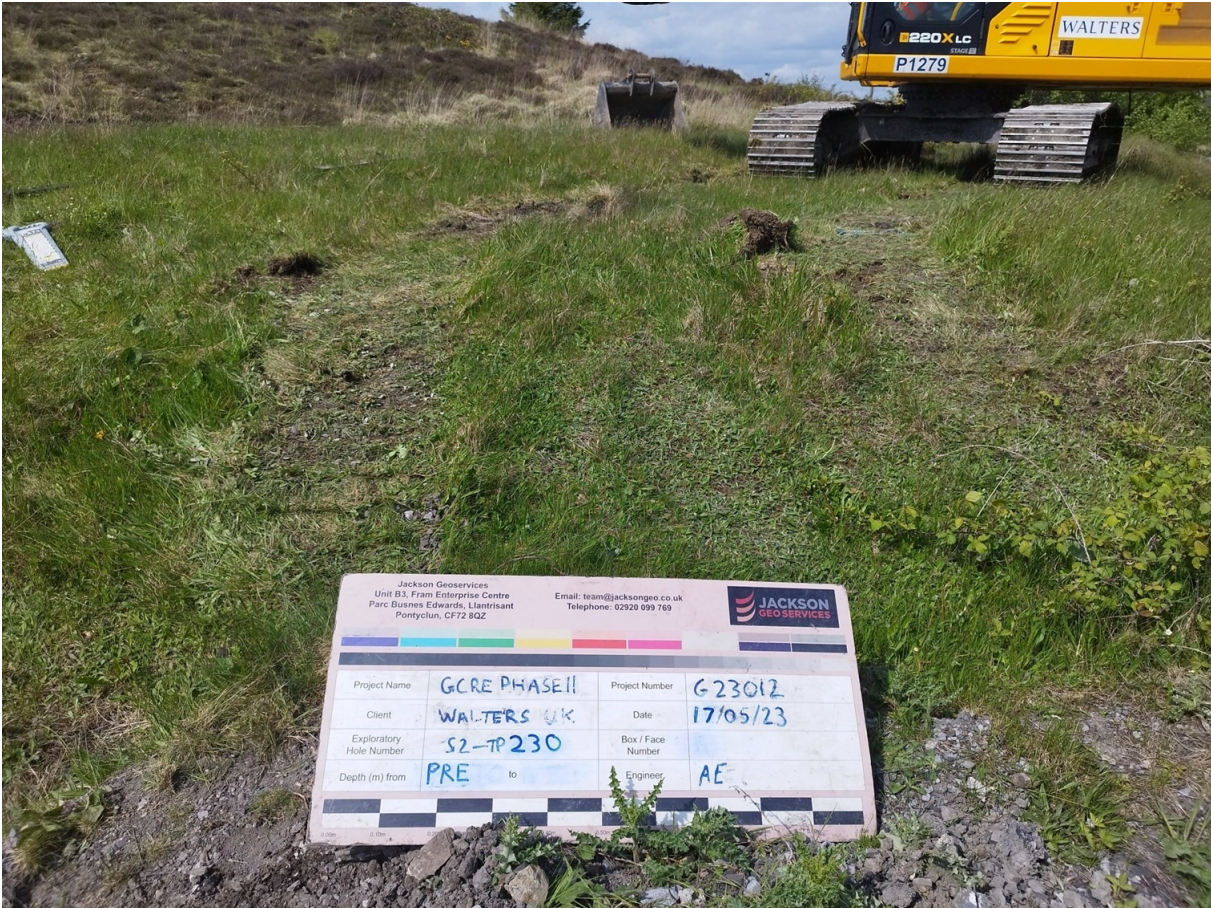
S2-TP230 Pre Excavation
