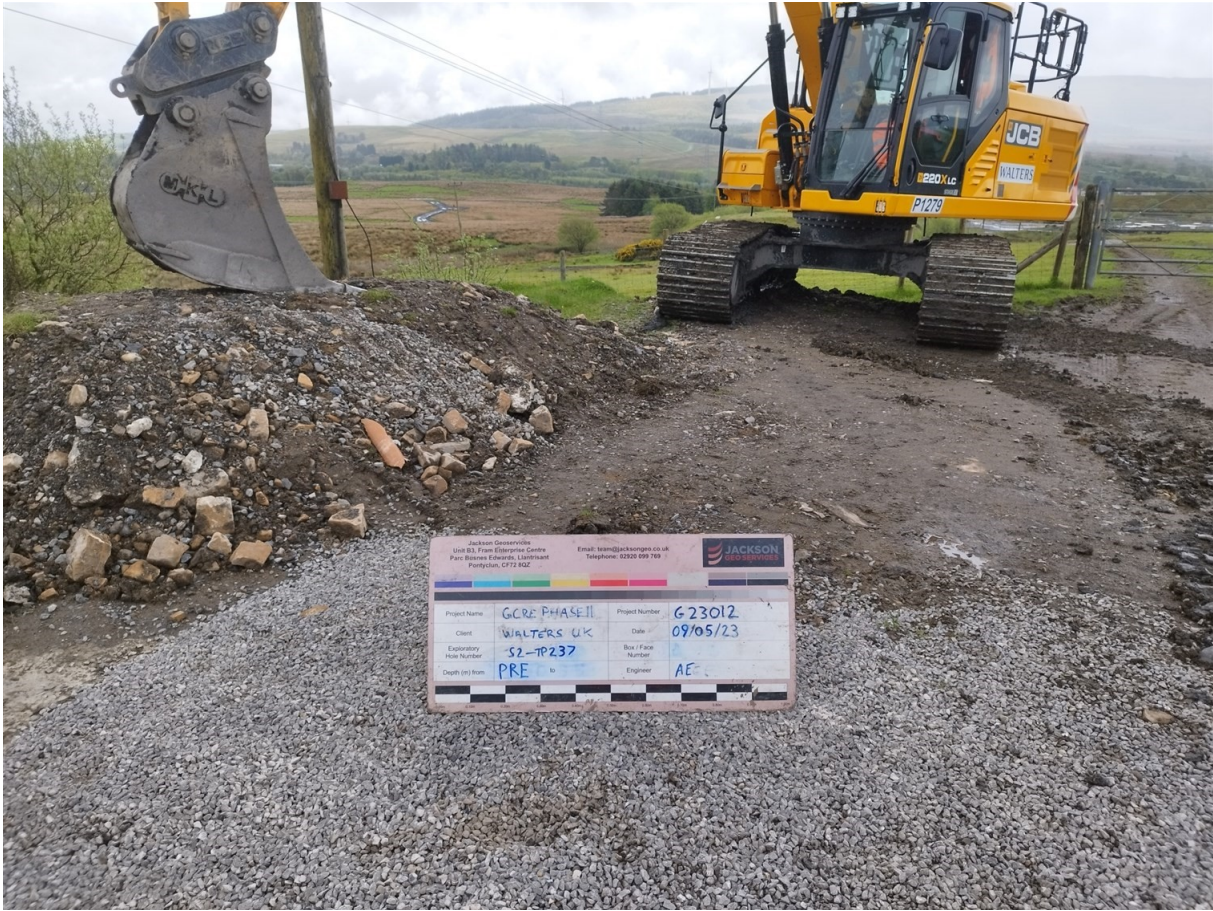
S2-TP237 Pre Excavation
