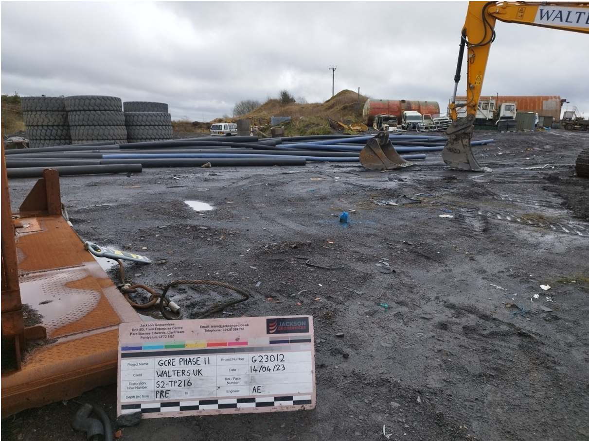
S2-TP216 Pre Excavation
