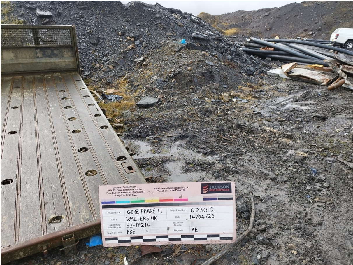
S2-TP214 Pre Excavation
