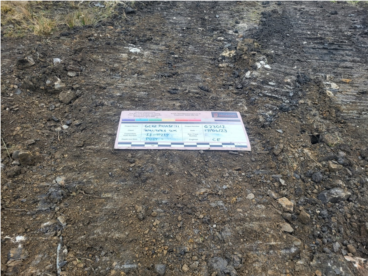
S2-TP217 Post Excavation
