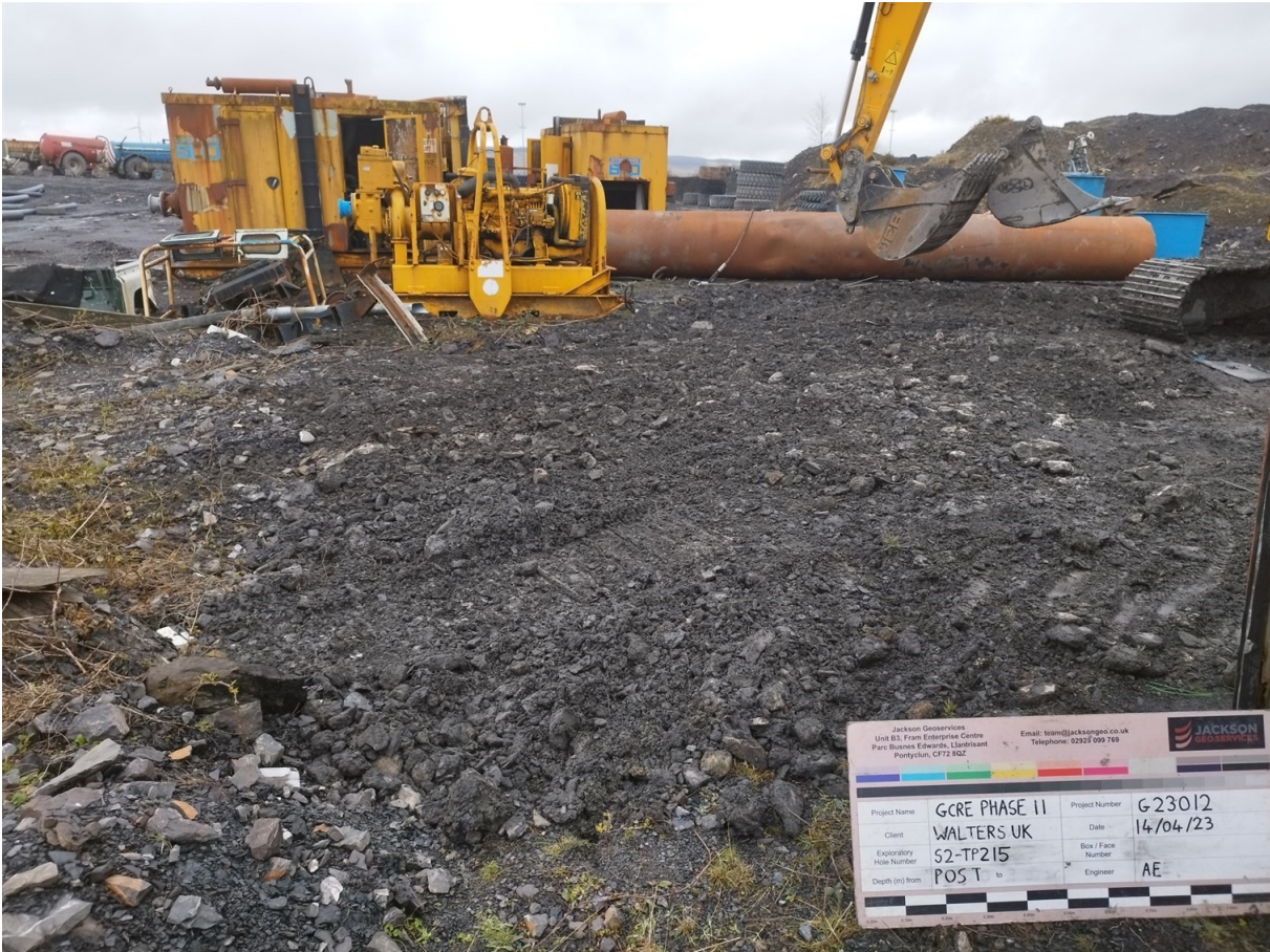
S2-TP215 Post Excavation
