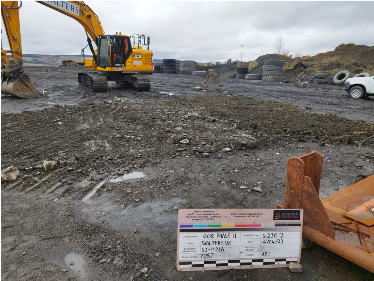
S2-TP216 Post Excavation
