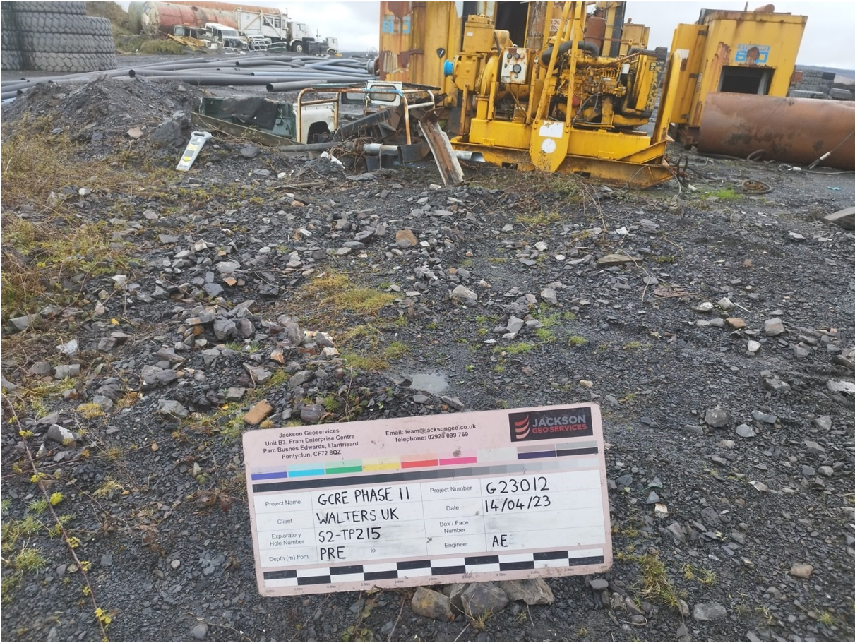
S2-TP215 Pre Excavation
