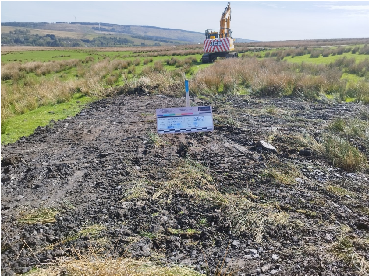
S2-TP209 Post Excavation
