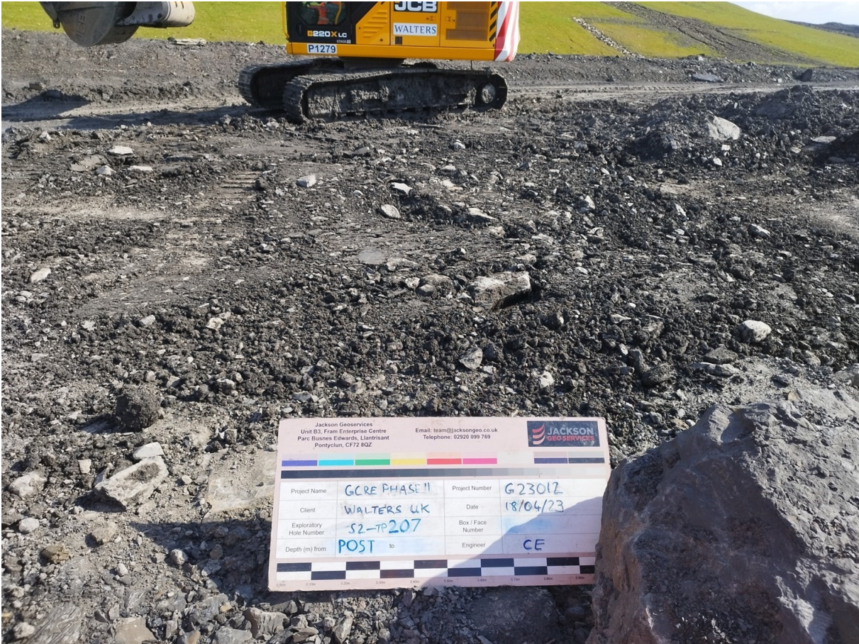
S2-TP207 Post Excavation
