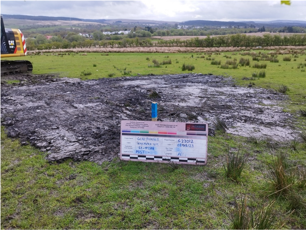
S2-TP208 Post Excavation
