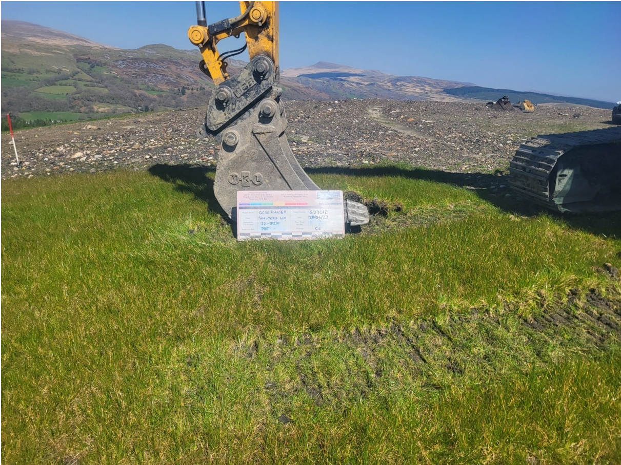
S2-TP210 Pre Excavation
