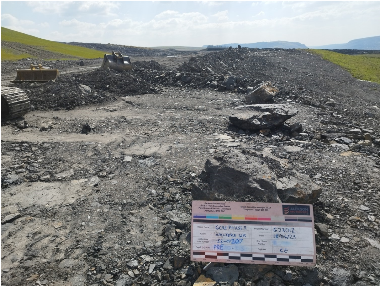
S2-TP207 Pre Excavation
