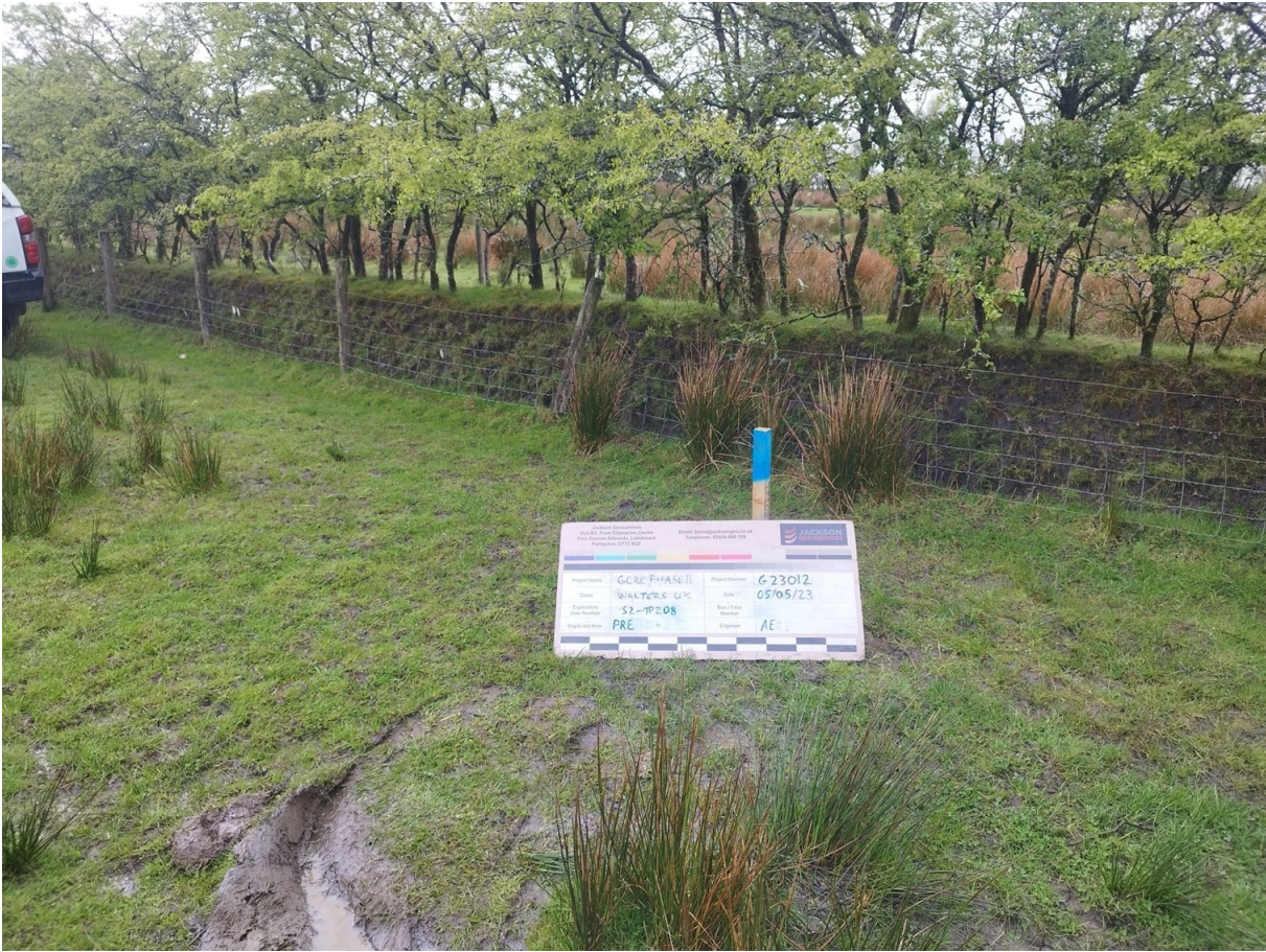
S2-TP208 Pre Excavation
