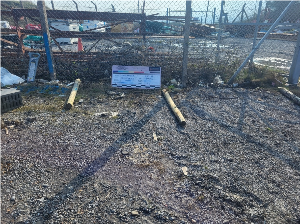
S2-TP223 Pre Excavation
