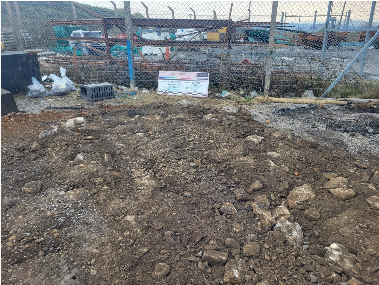
S2-TP223 Post Excavation
