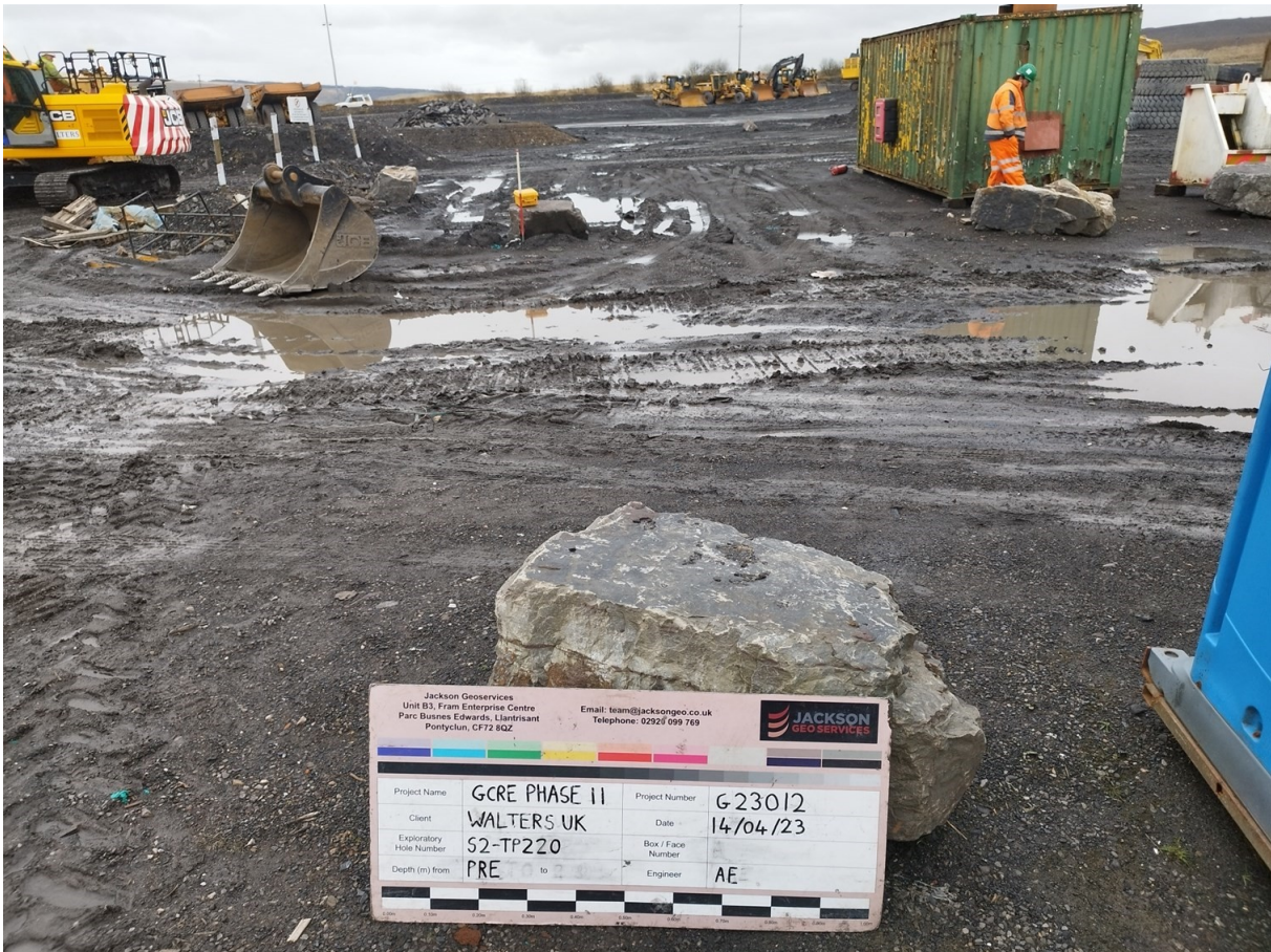
S2-TP220 Pre Excavation
