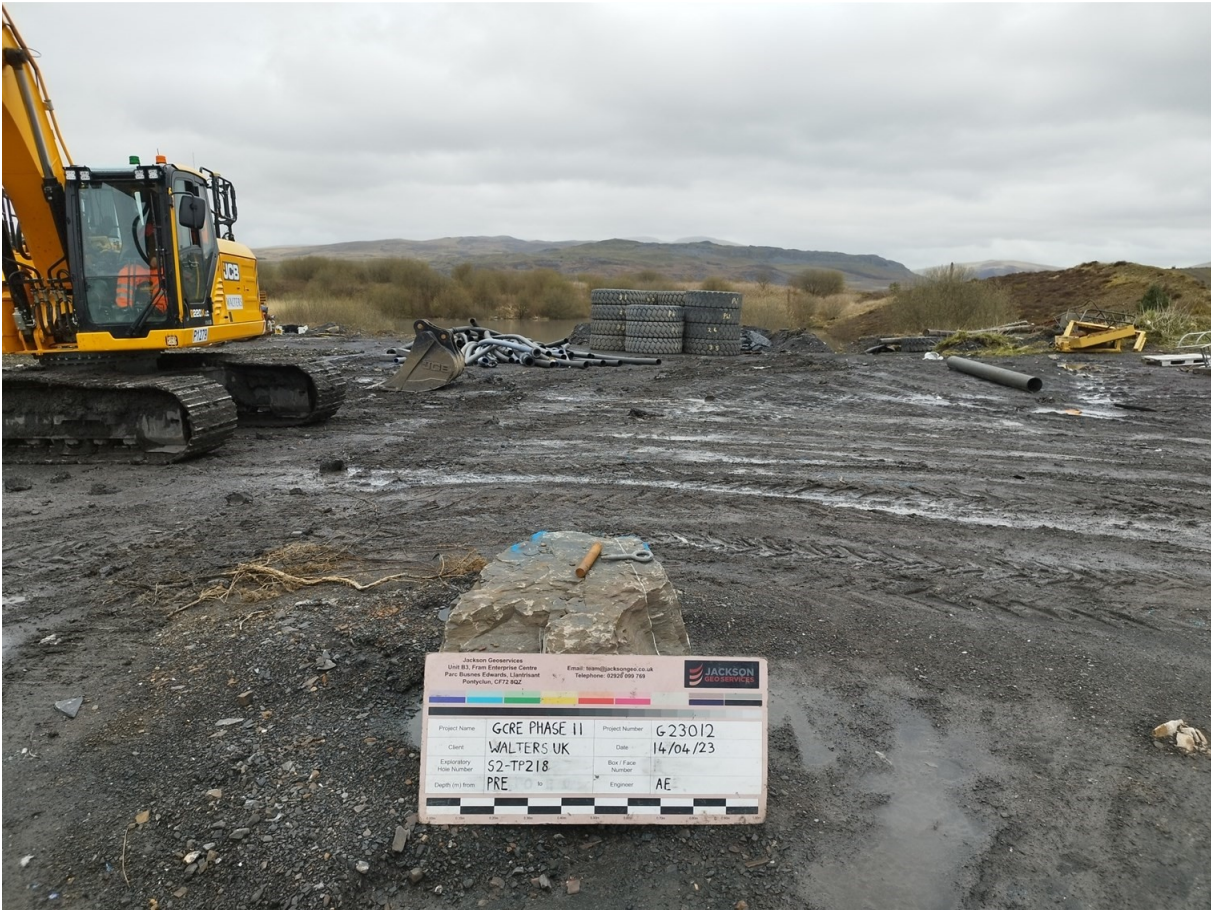
S2-TP218 Pre Excavation
