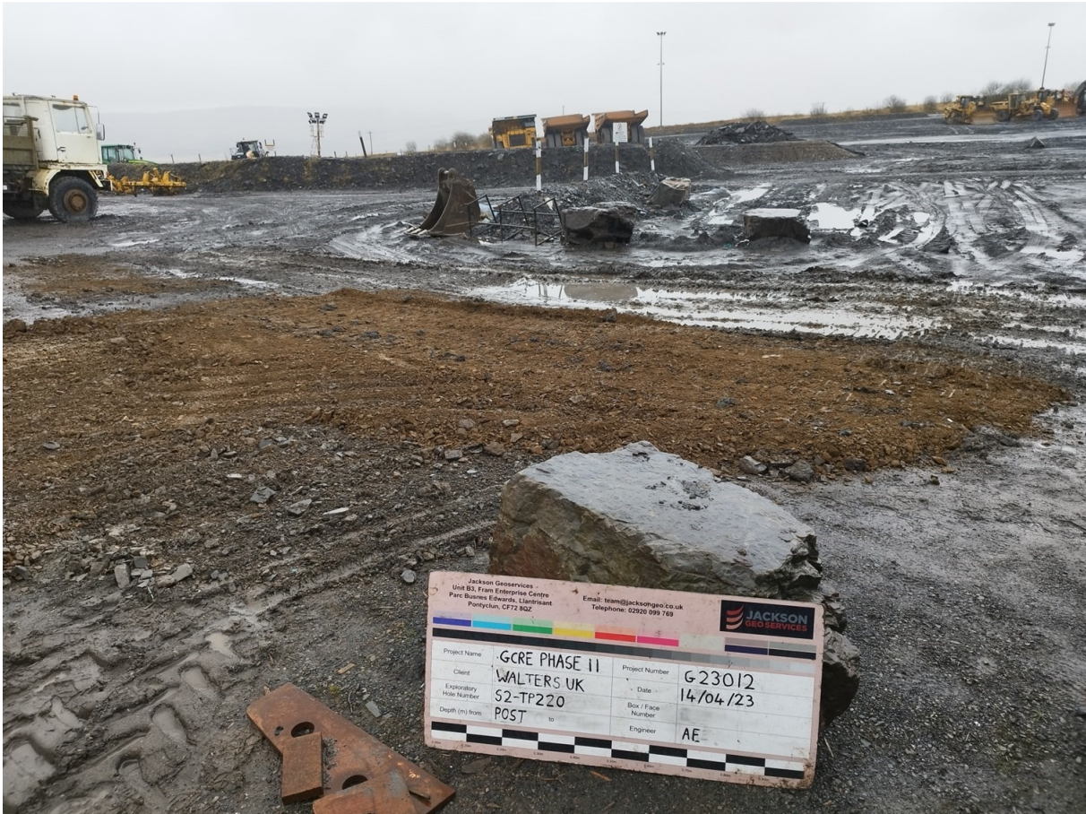
S2-TP220 Post Excavation
